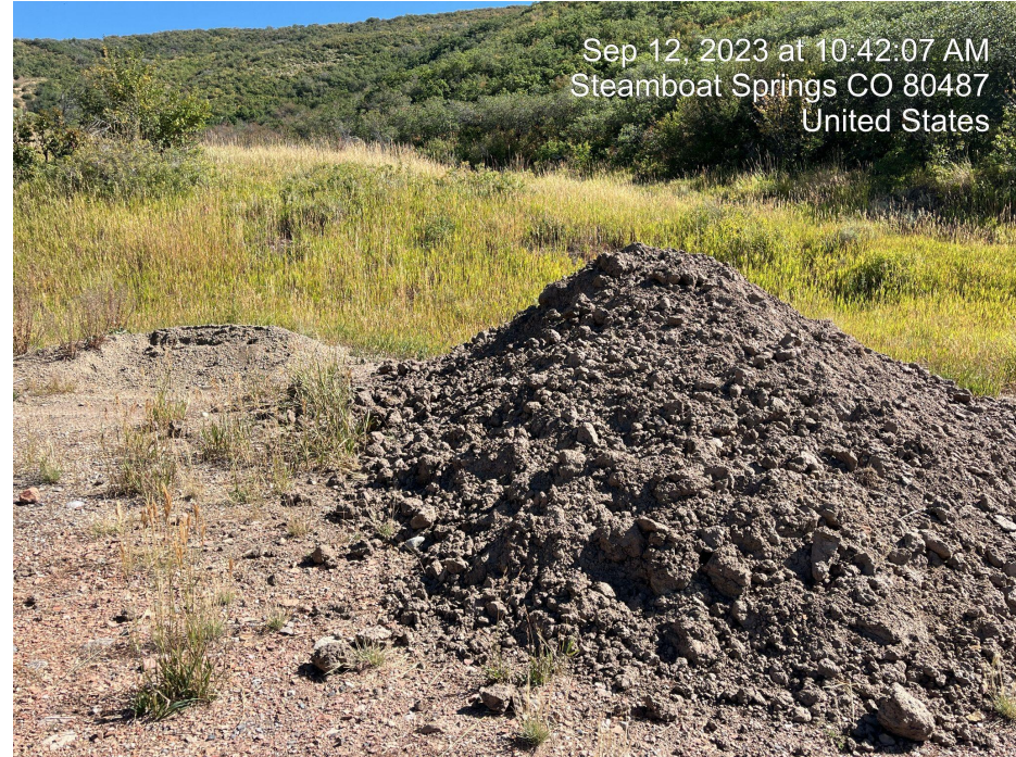
Photo 26. Soil stockpile observed without stormwater and erosion control BMPs per Rule 1002.c and 1002.f.
