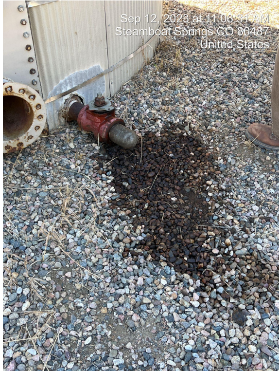
Photos 35 and 36: Photos taken from the Energy Investments tank battery facility on the northwest end of the Location. Active leak and stained soil around tank.
