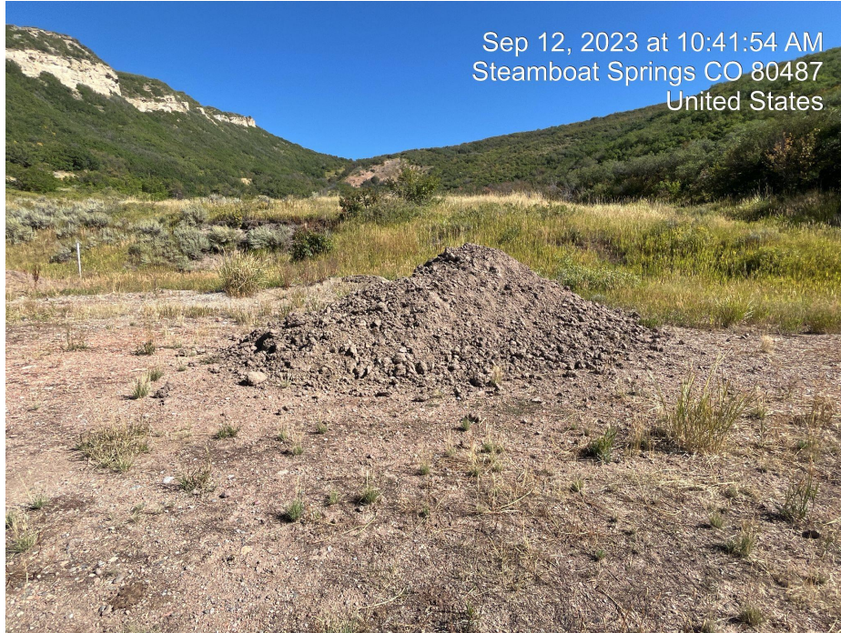
Photo 25. Soil stockpile observed without stormwater and erosion control BMPs per Rule 1002.c and 1002.f
