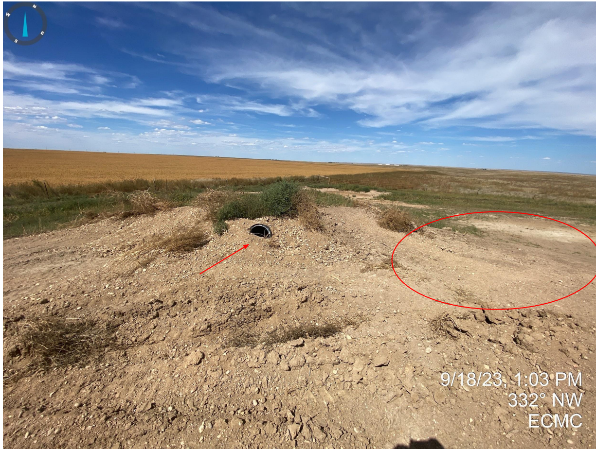
Photo 18. Taken near the northwest corner of the production areas. Stormwater control measures are partially buried and do not appear to be in properly functioning; no perimeter berm or other control measures observed right of the culvert (red circle).
