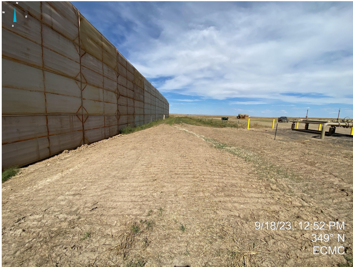
Photo 4. Taken near the east side of the location. Unstabilized soils were observed in the vicinity of midstream pipeline. The bare/exposed soils will need to be properly stabilized both temporarily (before interim reclamation activities) and also for long term stabilization to prevent wind and water erosion degradation.
