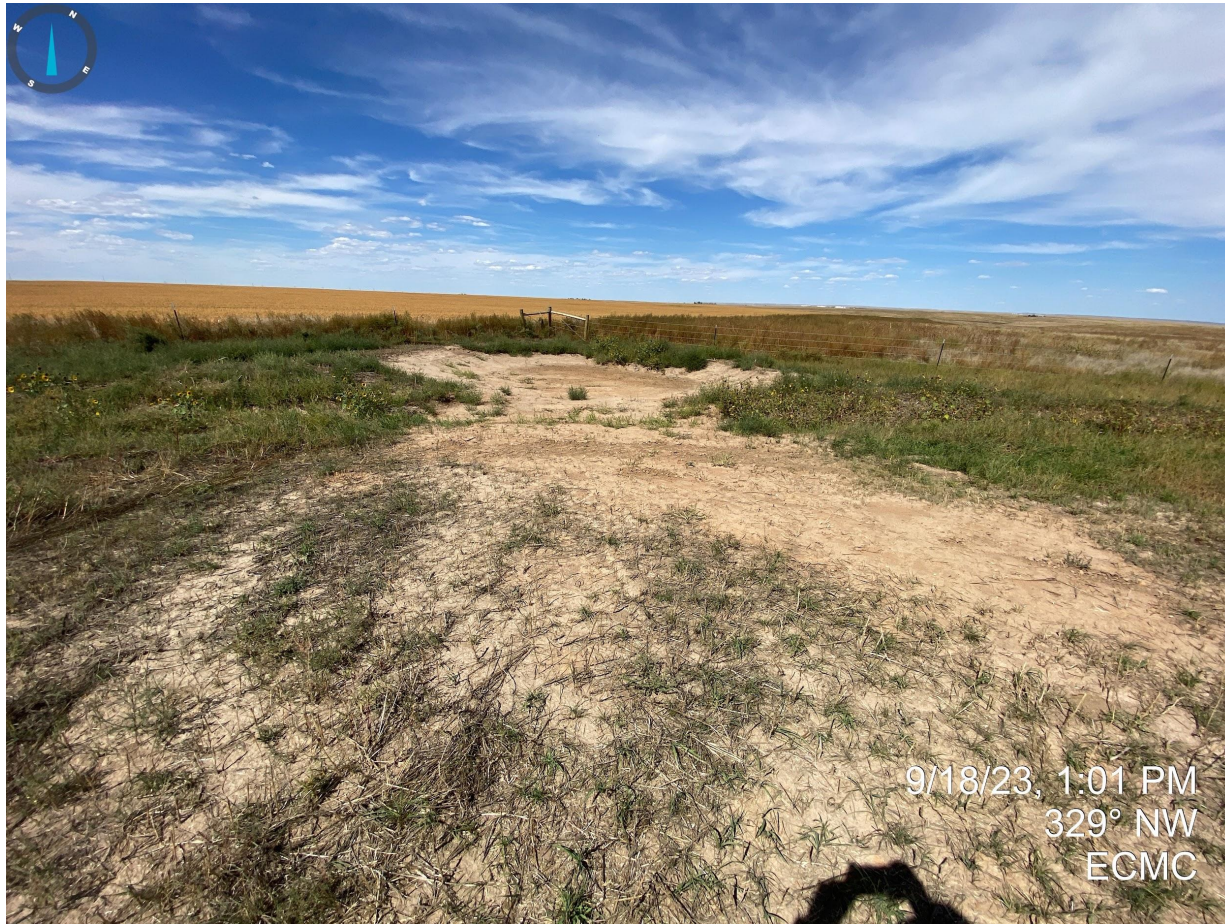
Photo 15. Facing towards the northwest corner of the location. Previous inspections documented that the sediment trap pictured here appeared to be inadequate in size to control stormwater from a location of this size. Previous corrective actions required the Operator to repair/install adequate stormwater control measures; nothing appears to have been completed as of this inspection.
