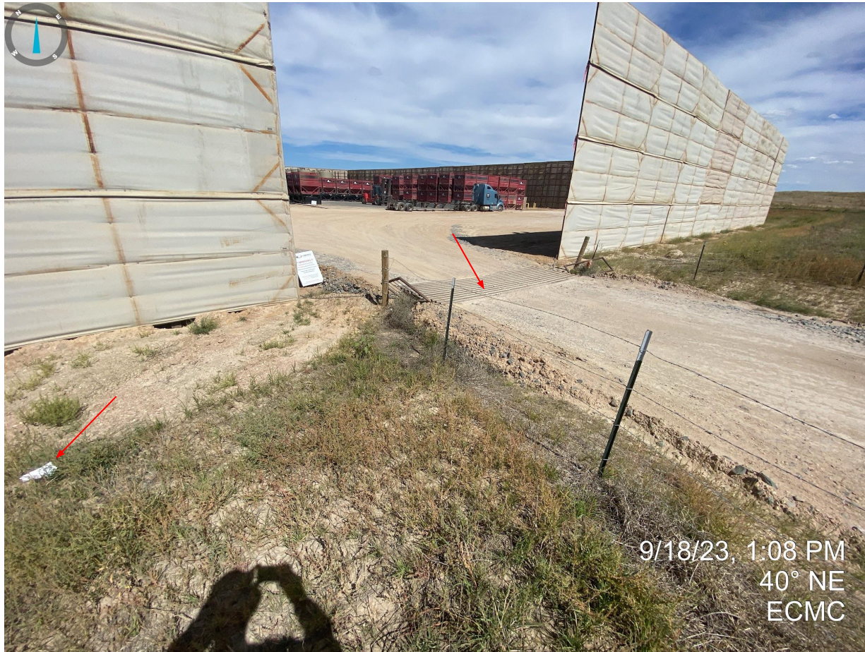
Photo 23. Taken near the entrance to the location. Photo illustrates trash and a cattle guard that requires maintenance as sediment is beginning to fill in.
