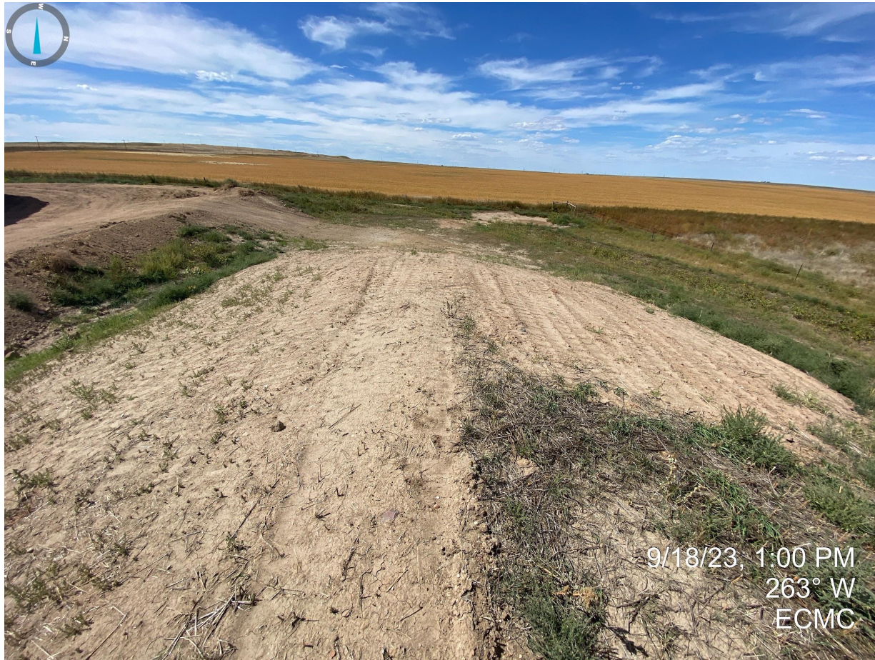
Photo 13. Taken from the western portion of the topsoil stockpile. Photo illustrates that the topsoil stockpile is not properly stabilized with evidence of bare/exposed soils.
