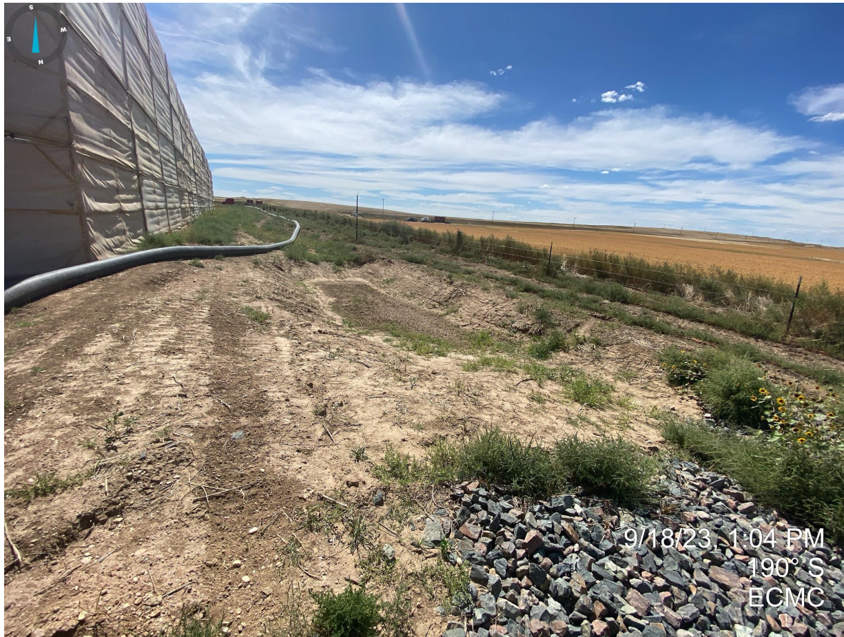
Photo 20. Taken from the west side of the location. Photo illustrates that areas not needed for active drilling do not comply with Rule 1002.c. with evidence of undesirable vegetation (e.g. russian thistle and kochia) and bare/exposed soils.
