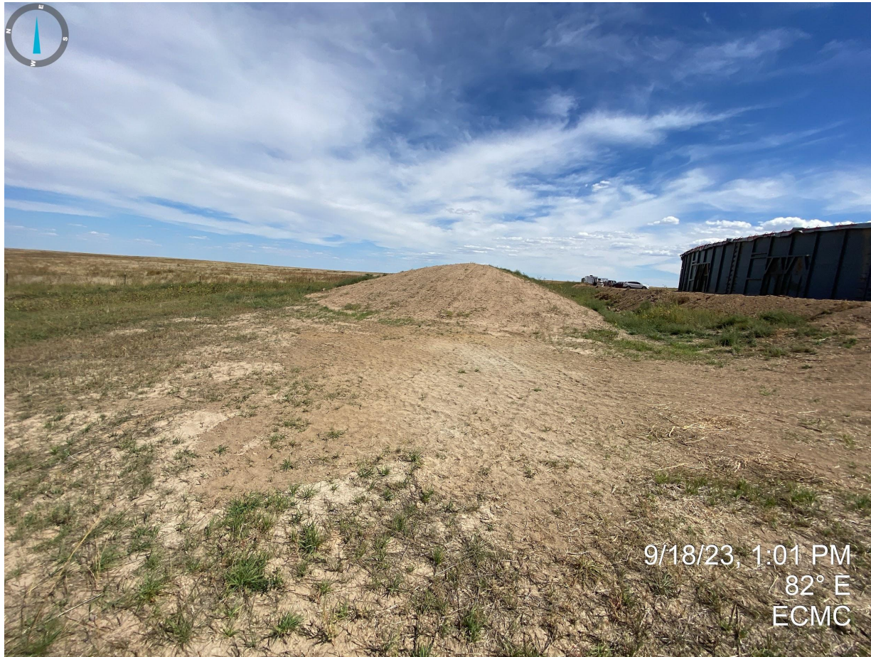
Photo 14. Taken west of the topsoil stockpile. Photo illustrates that the topsoil is not properly stabilized (e.g. exposed soils) and there are no apparent stormwater control measures/BMPs observed to prevent topsoil from erosion degradation and exiting off into the sediment trap (outside of frame to the left in photo).
