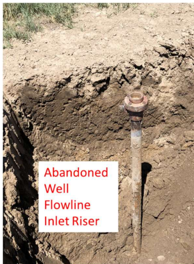
Figure 5- The Abandoned Well Flowline Inlet Riser
