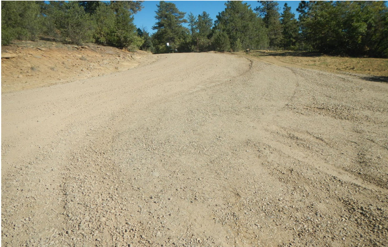
Photo 1. Facing north at the beginning of the main road. Additional gravel has been applied to areas of the road.
