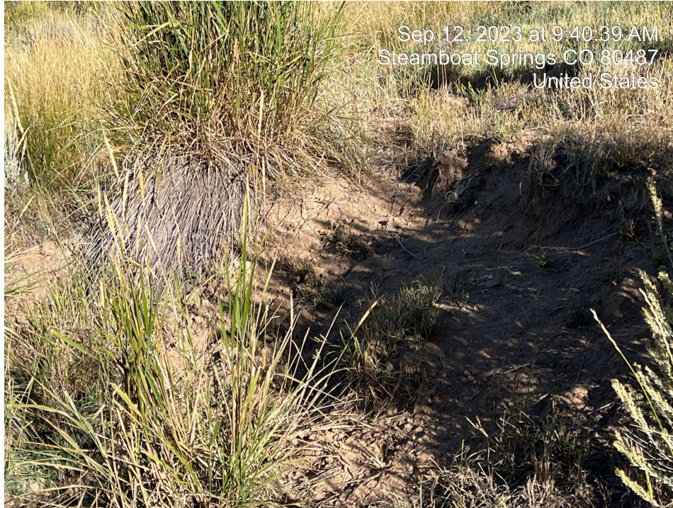
Photo 18. Observed gully erosion on fill slope.
