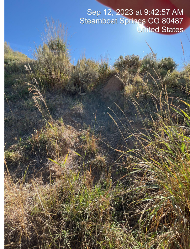
Photo 19. Observed gully erosion on fill slope.
