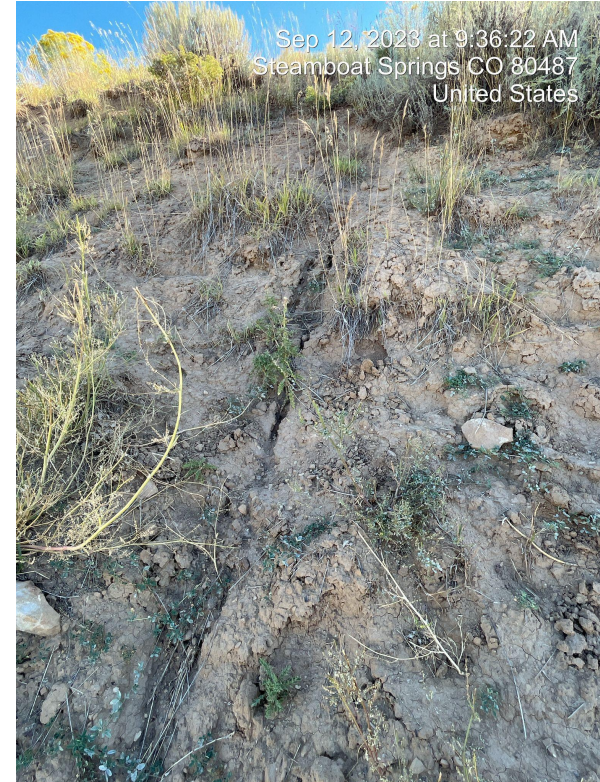
Photo 21. Observed erosion occurring on cut slope.
