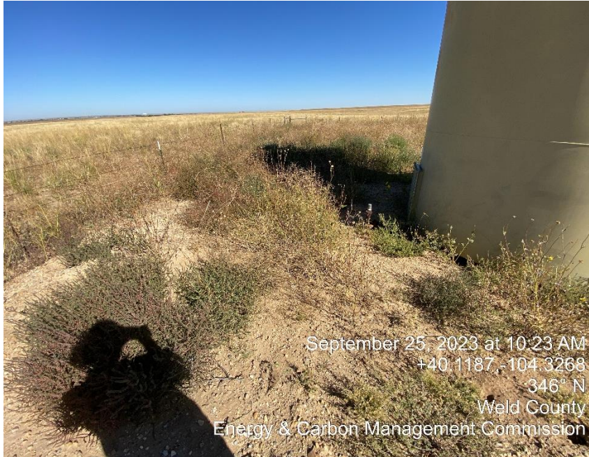
Weathered Berm & Overgrown Vegetation
