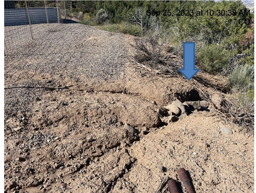
Photo # 566 BMP needs maintenance (N/NE area of location)
