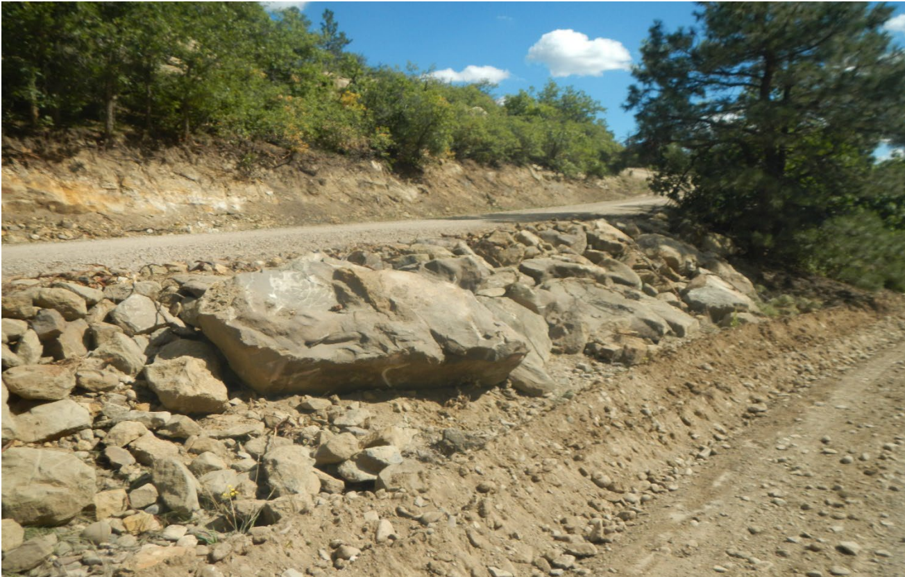
Photo 2. The road side has been stabilized with large rock rip/rap.
