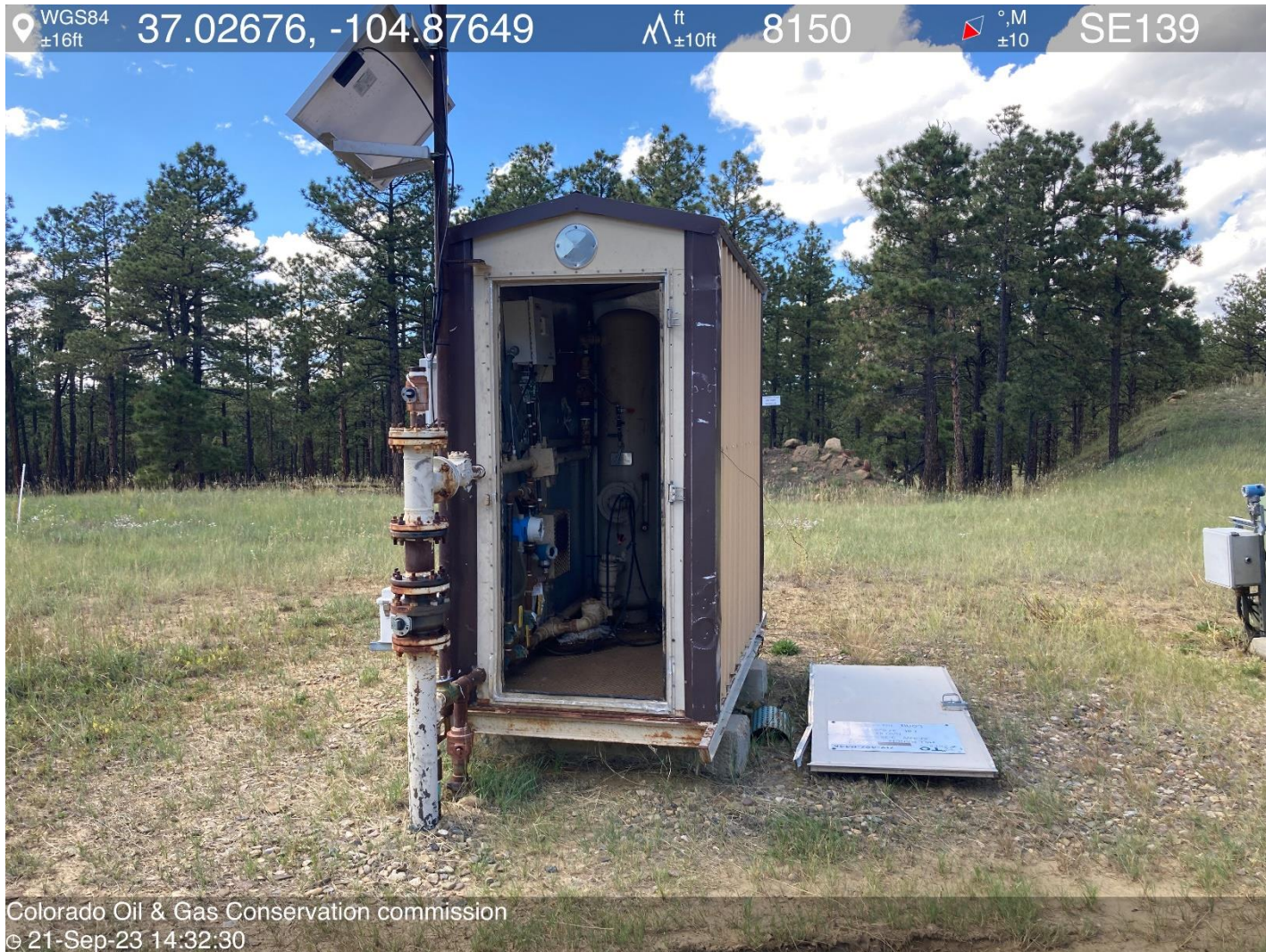
PHOTO 4: METER HOUSE DOOR WITH WELL SIGN IS DETACHED FROM METER HOUSE AND LYING ON THE GROUND. POST SIGN PER RULE 605 AND REPAIR OR REMOVE DOOR FROM LOCATIO PER RULE 606. CA DATE 10-26-2023.
