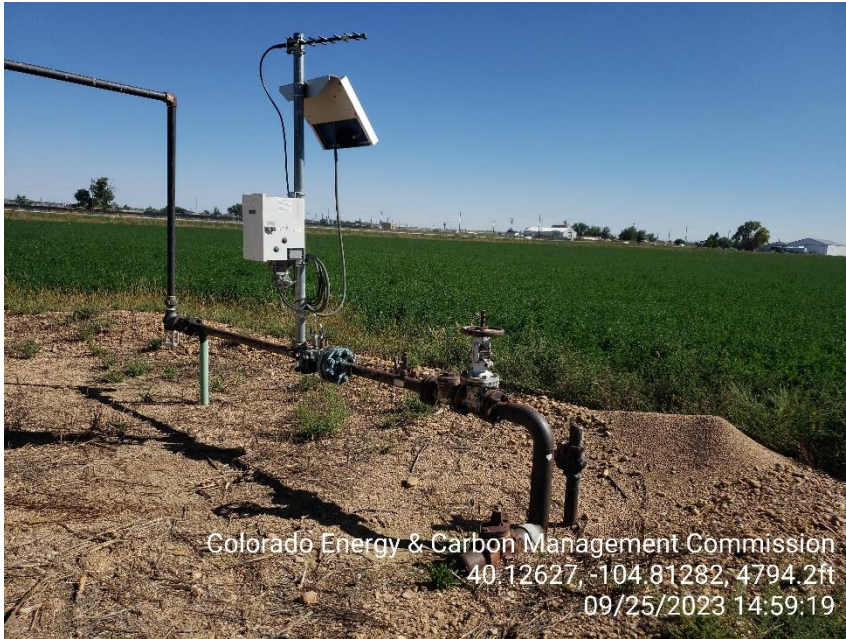
Photo7 Gas Meter Run.
