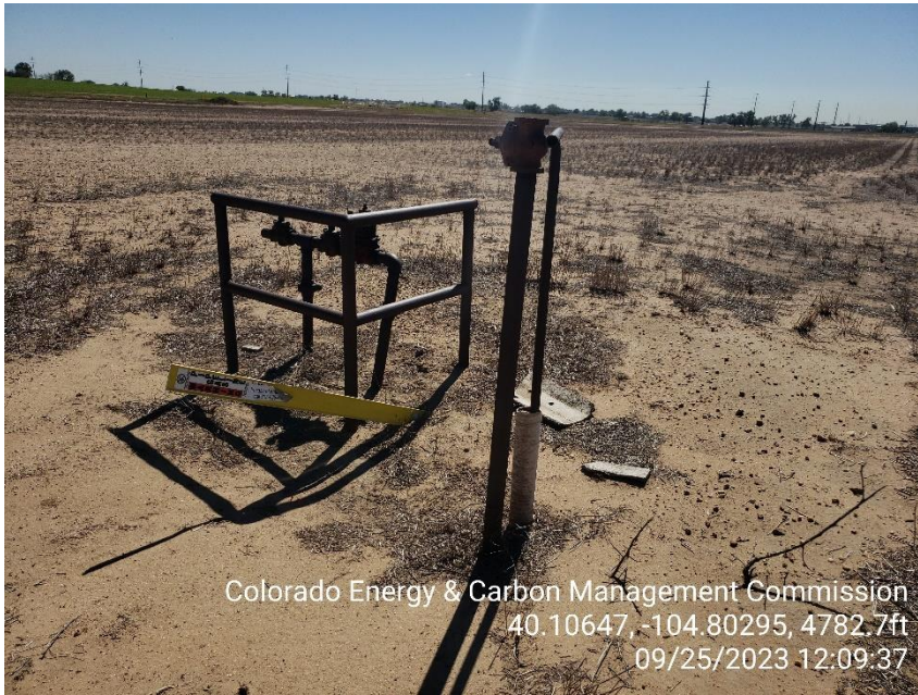
Photo 17 Marked flow line not LOTO.
