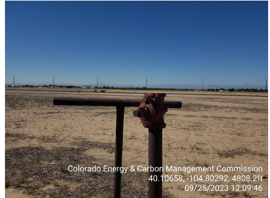
Photo 18 Marked flow line not LOTO.
