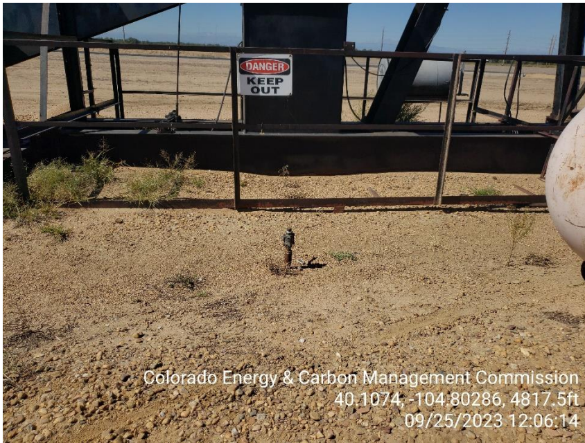
Photo 9 Unused flow line with ball valve not LOTO .
