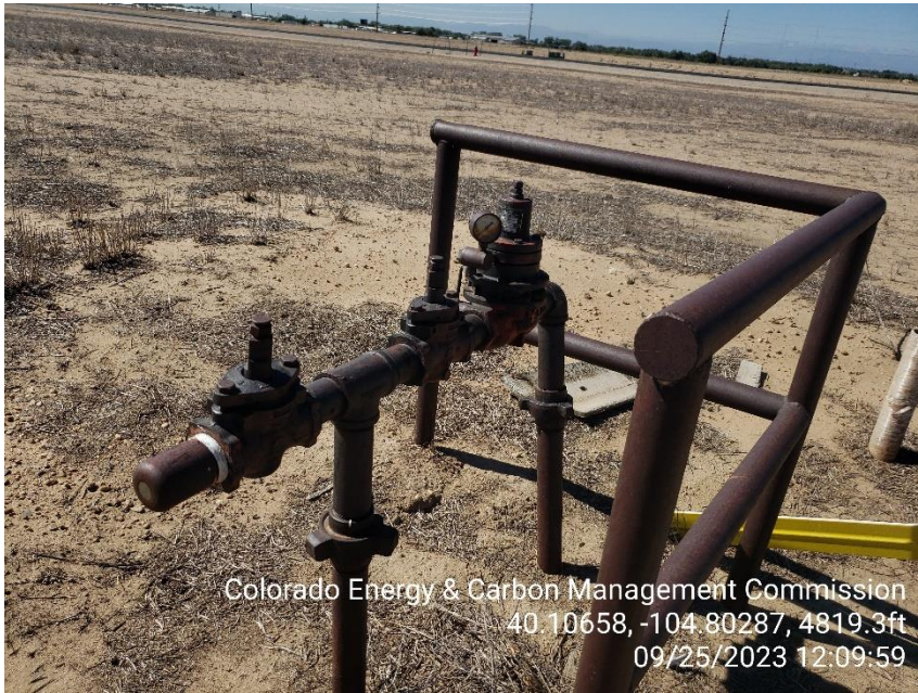
Photo 19 Marked flow line not LOTO.
