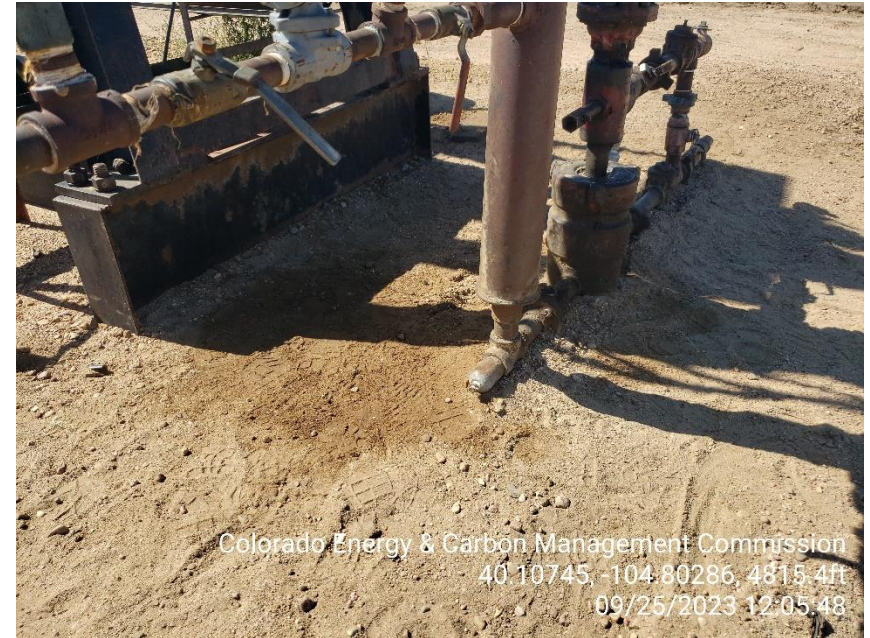
Photo 12 Stained soil around the WH and pump jack base.
