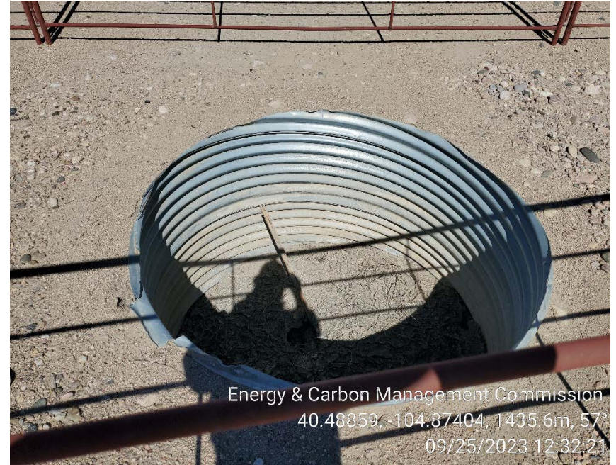
Cellar ring on wellhead site
