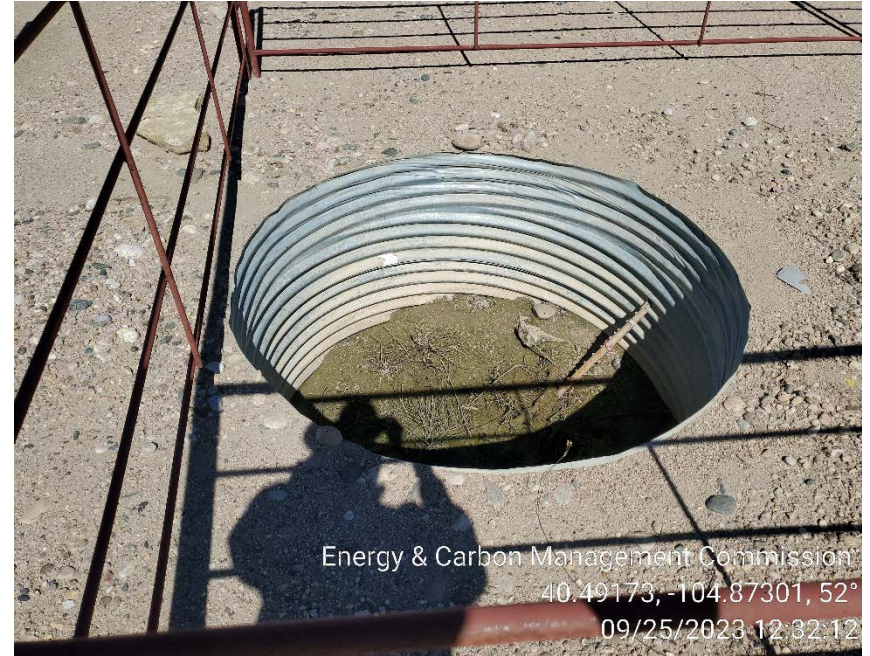
Cellar ring on wellhead site
