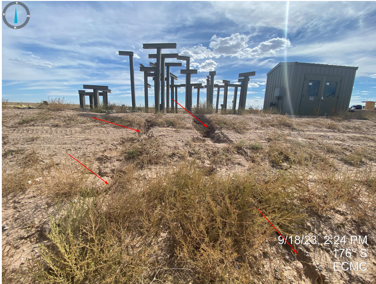
Photo 11. Continued from Photo 10; erosion degradation (e.g. gullying) pictured.
