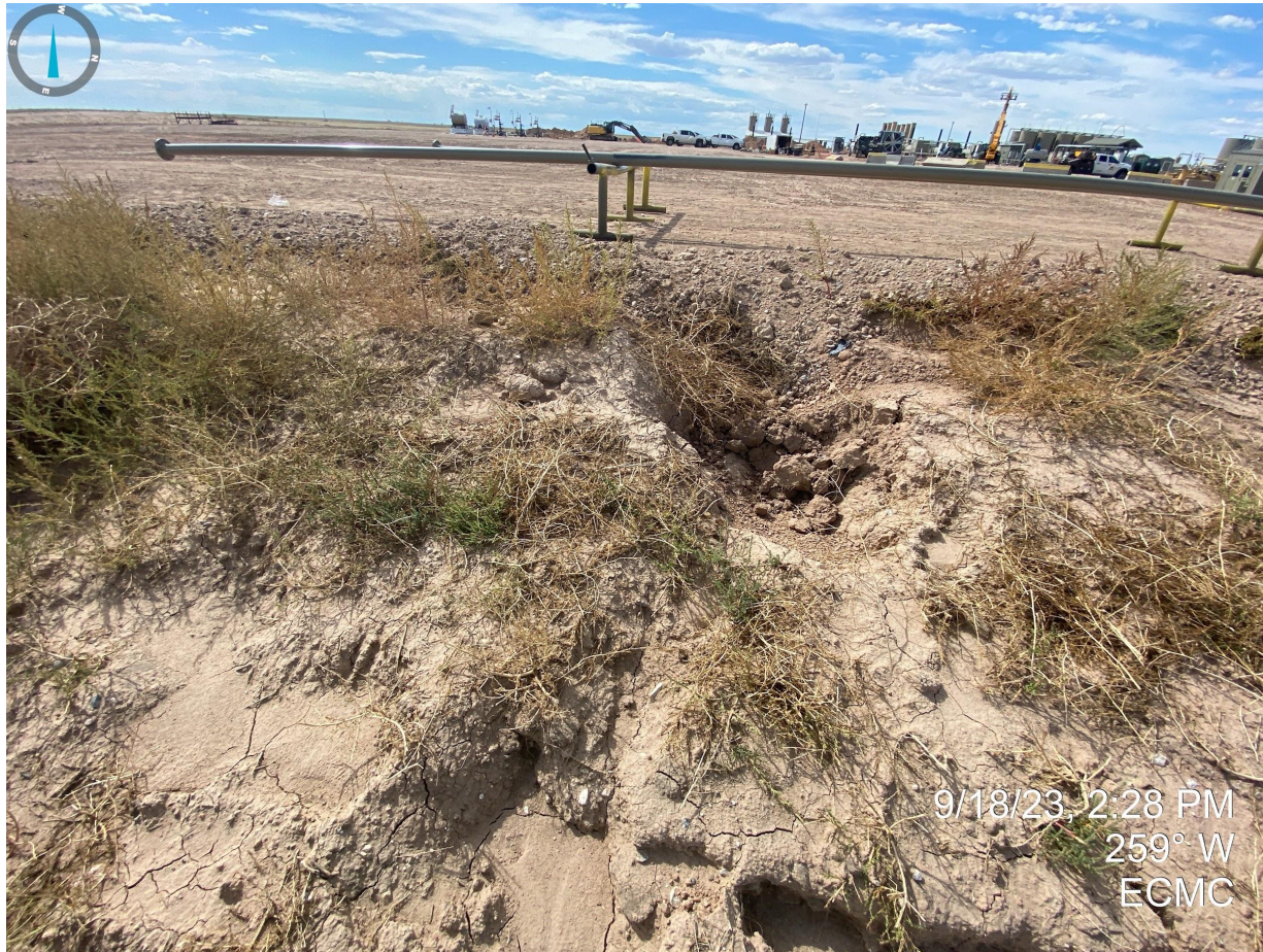
Photo 15. Taken from the eastern side of the production pad. Erosion degradation and undesirable vegetation observed.
