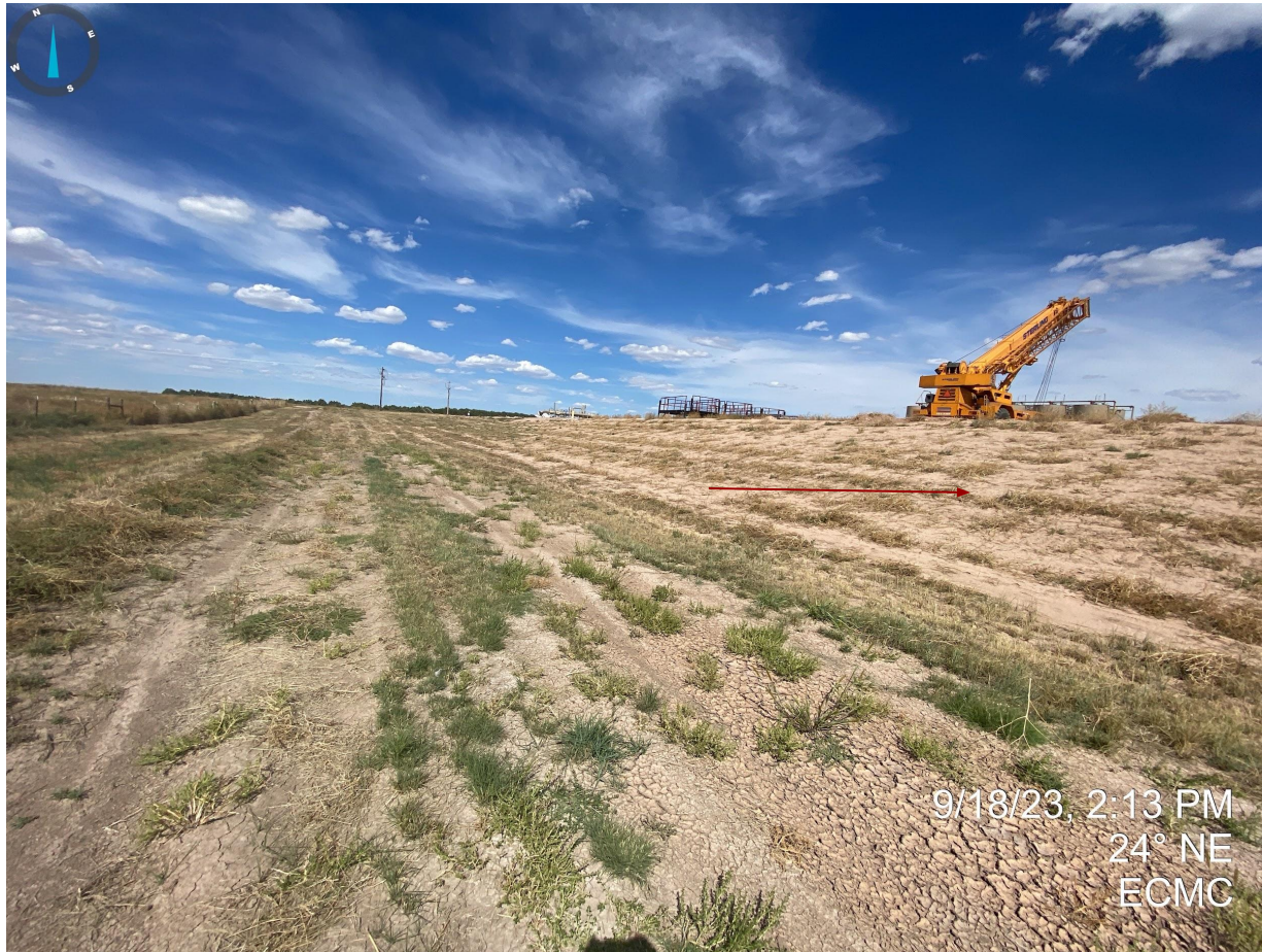
Photo 1. Taken from the western portion of the location. Portions of the production areas do not appear to be properly stabilized with evidence of bare and exposed soils. Additionally, undesirable vegetation (e.g. kochia and russian thistle) was observed throughout and will need to be properly managed for.
