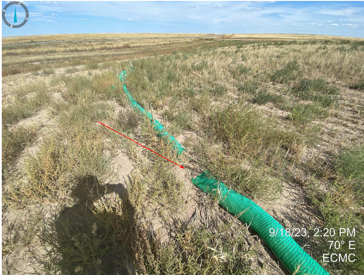
Photo 5. Taken from the northwestern portion of the topsoil stockpile. Photo illustrates that stormwater control measures (e.g. filtrex) are beginning to degrade and fill with sediment.
