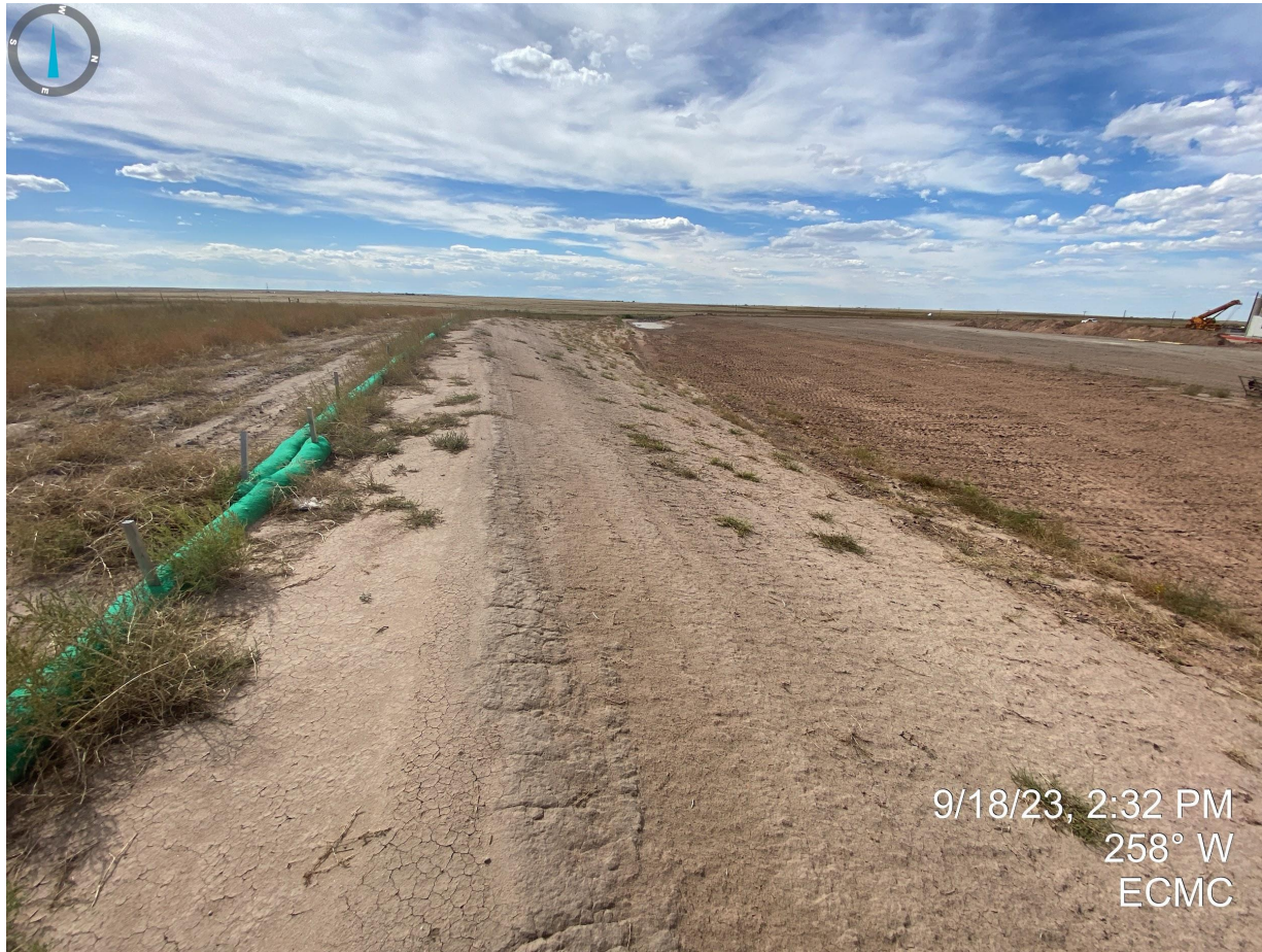
Photo 26. Taken from the center/southern portion of the location. Stormwater control measures do not appear to be properly stabilized with evidence of bare and exposed soils.
