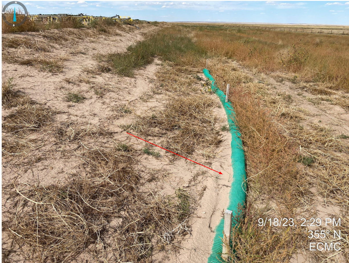
Photo 19. Taken from the eastern side of the production area. Stormwater control measures require maintenance to be properly functioning.
