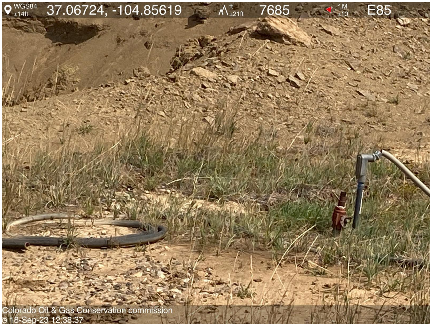
PHOTO 4: UNUSED RISER NOT MARKED OR PLUGGED. MARK AND PLUG OR USE UNUSED EQUIPMENT PER RULE 606. CA DATE 10-25-2023.
