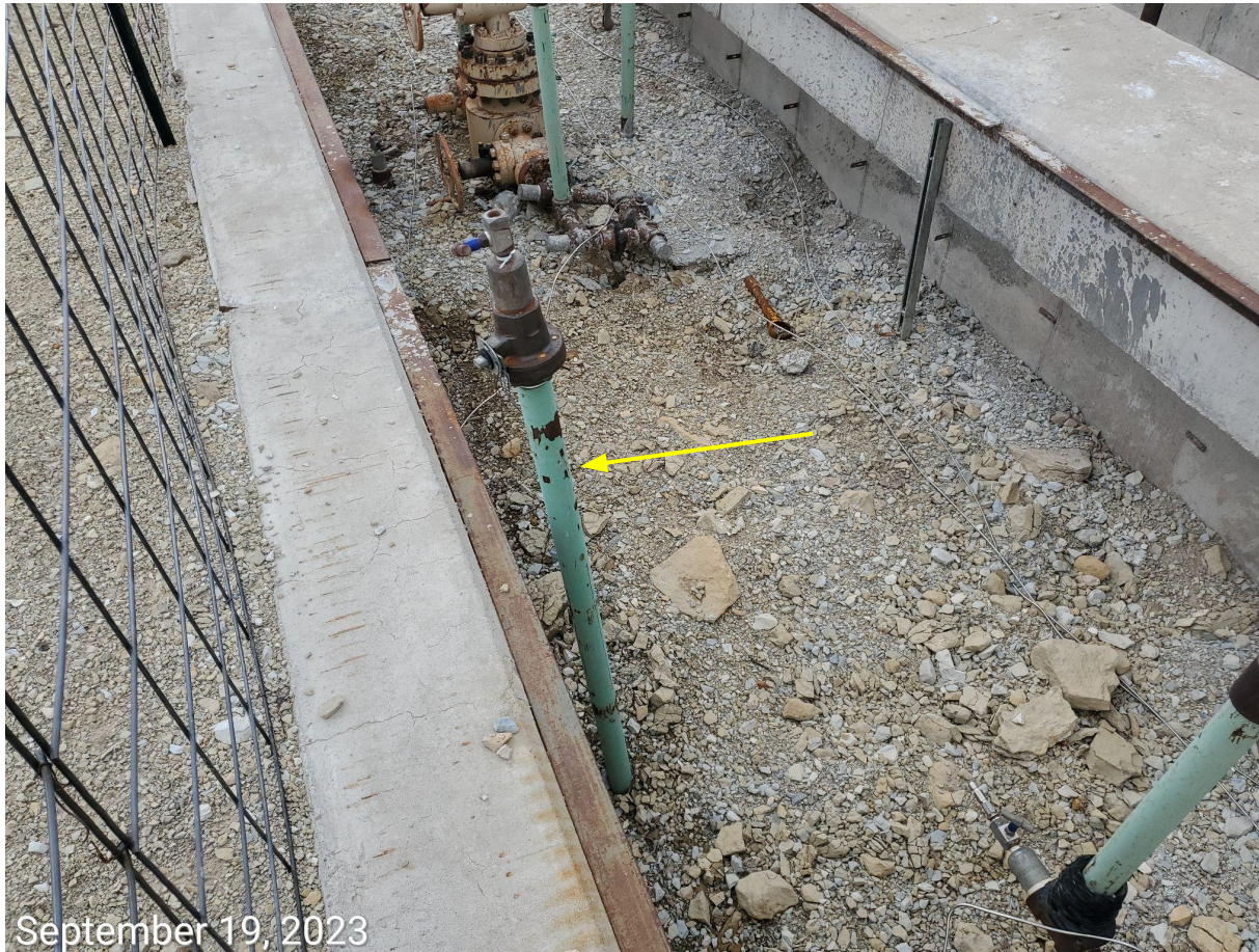
Photo 3: Photo taken from the Cascade Creek #697-09-10A well; well was PA 9/10/2021. Photo shows riser remaining.
