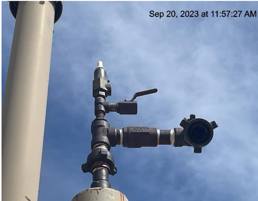
Photo # 9979 Open ended pipe on separator/wildlife hazard
