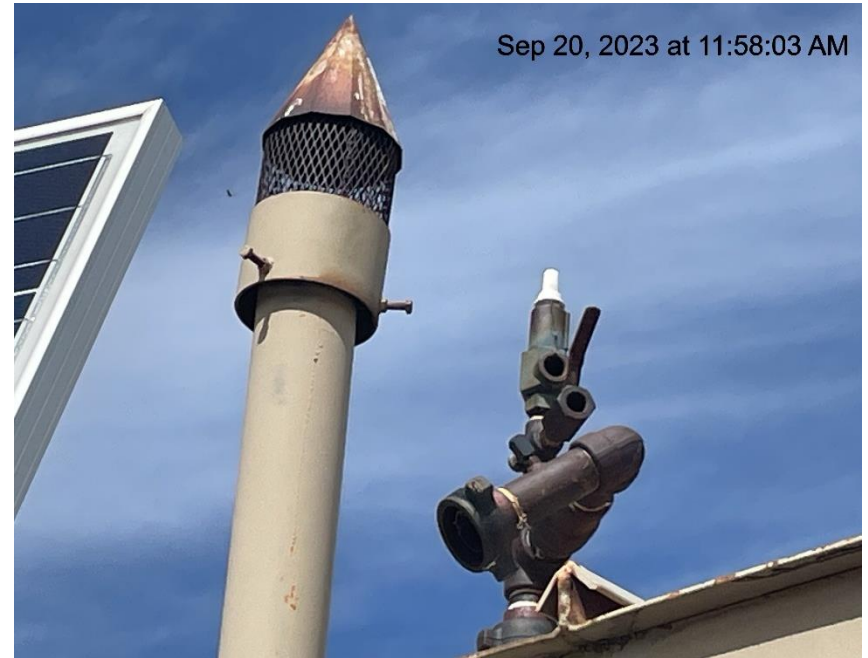
Photo # 9980 Open ended pipe on separator/wildlife hazard
