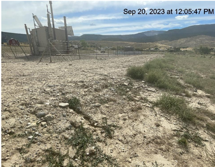
Photo # 10010 Erosion & transport of sediment off location & into vegetation/insufficient BMP's
