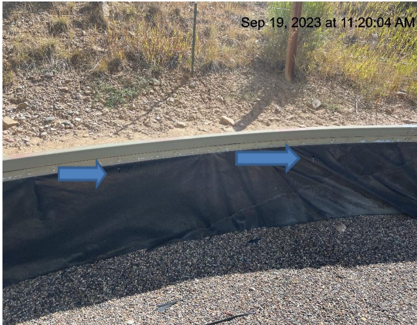
Photo # 9857 Holes in secondary containment liner
