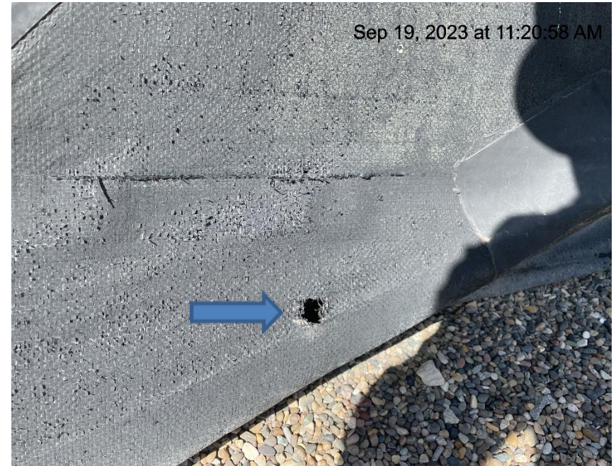
Photo # 9863 Hole in secondary containment liner
