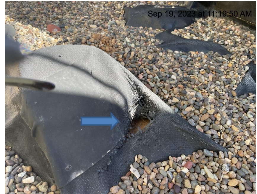
Photo # 9855 Hole in containment liner
