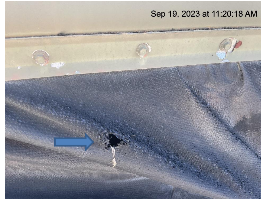
Photo # 9859 Hole in secondary containment liner
