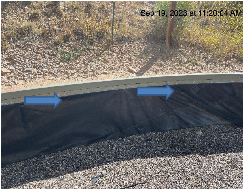
Photo # 9857 Holes in secondary containment liner
