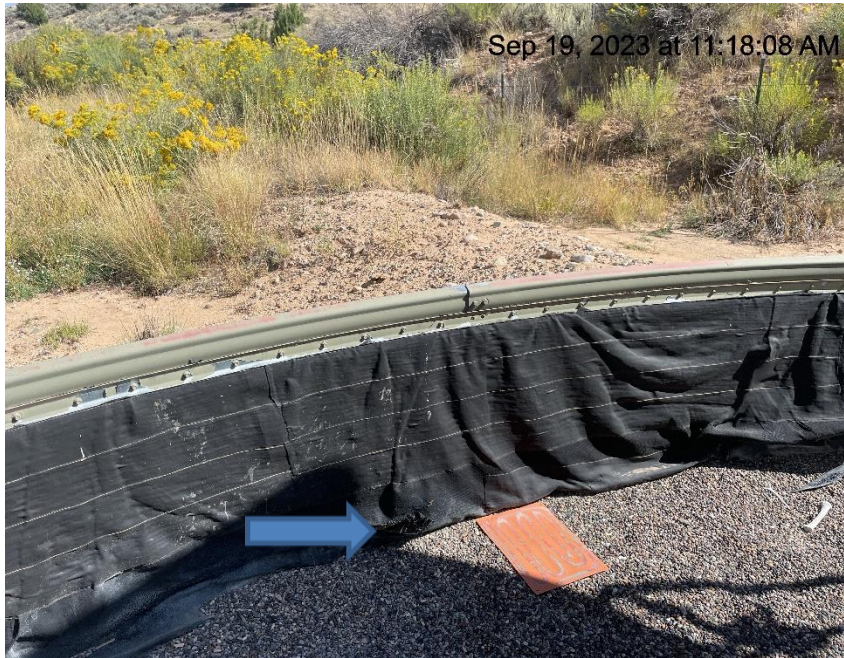
Photo # 9852 Holes in containment liner
