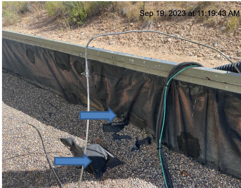
Photo # 9854 Holes in containment liner
