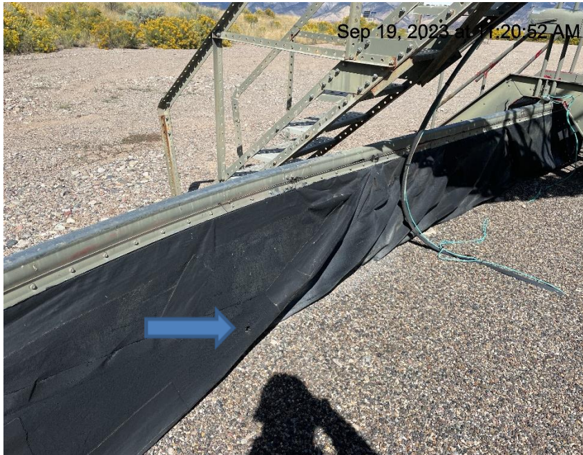
Photo # 9862 Holes in secondary containment liner
