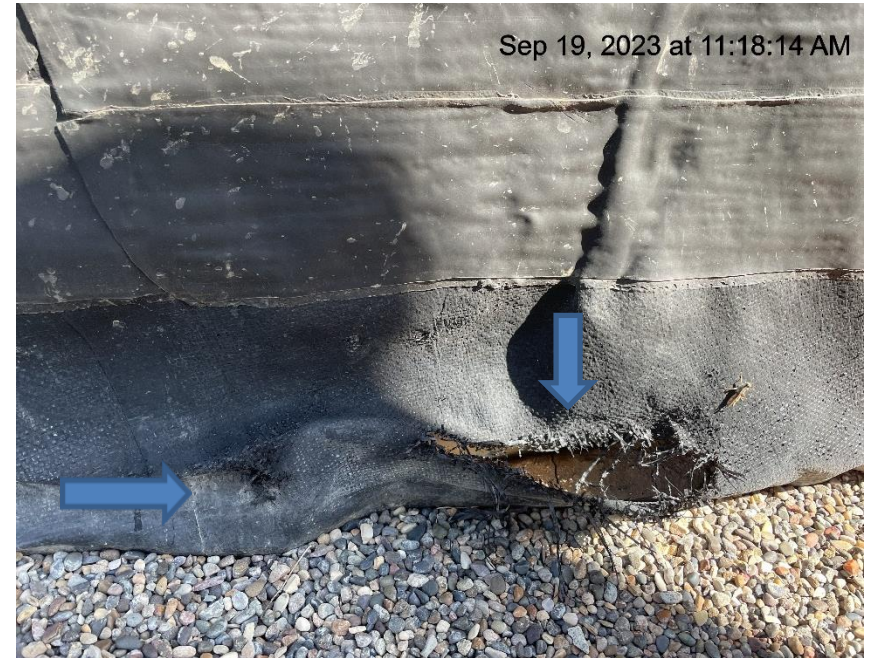
Photo # 9853 Holes in containment liner
