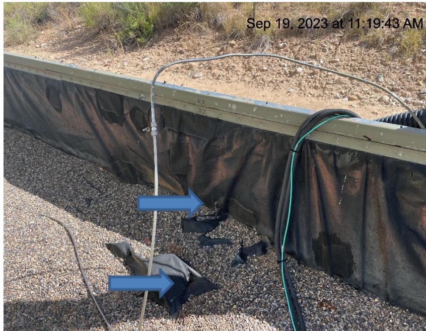
Photo # 9854 Holes in secondary containment liner
