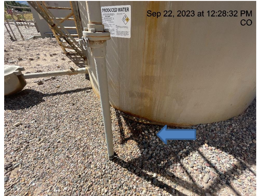
Photo # 469 Stained soils & gravel inside tank battery secondary containment/fluid running down side of tank
