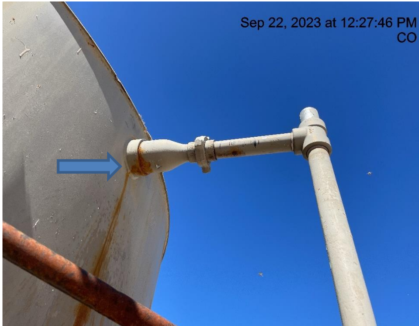
Photo # 463 Fluid leaking from swedge on tank
