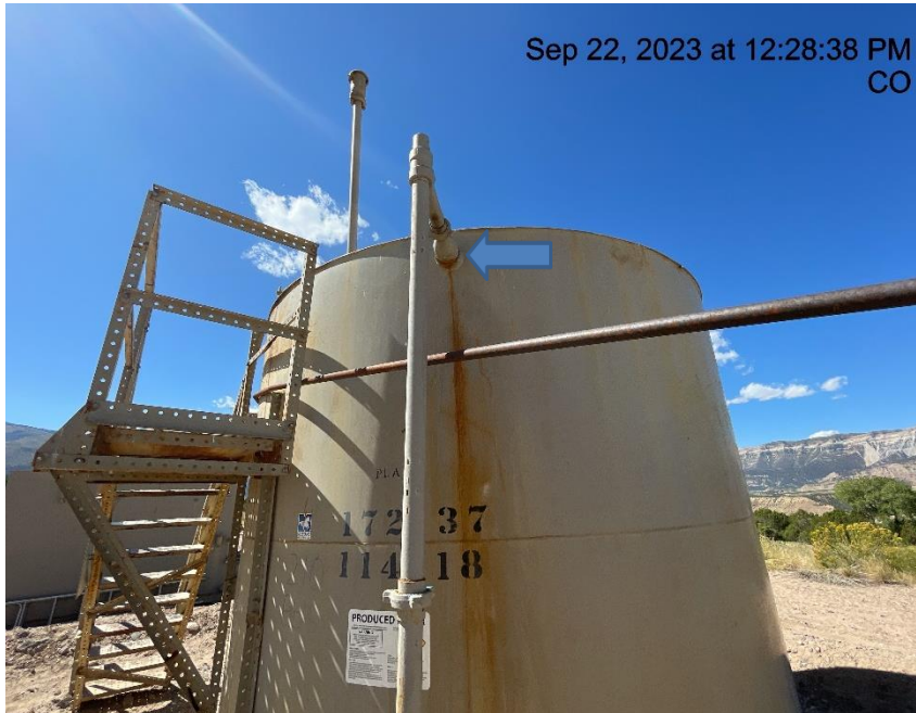
Photo # 470 Swedge leaking & fluid running down tank
