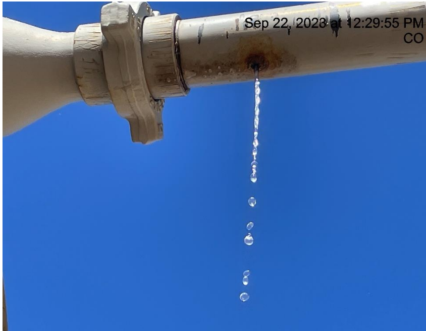
Photo # 489 Hole in production tank flowline & fluid leaking out
