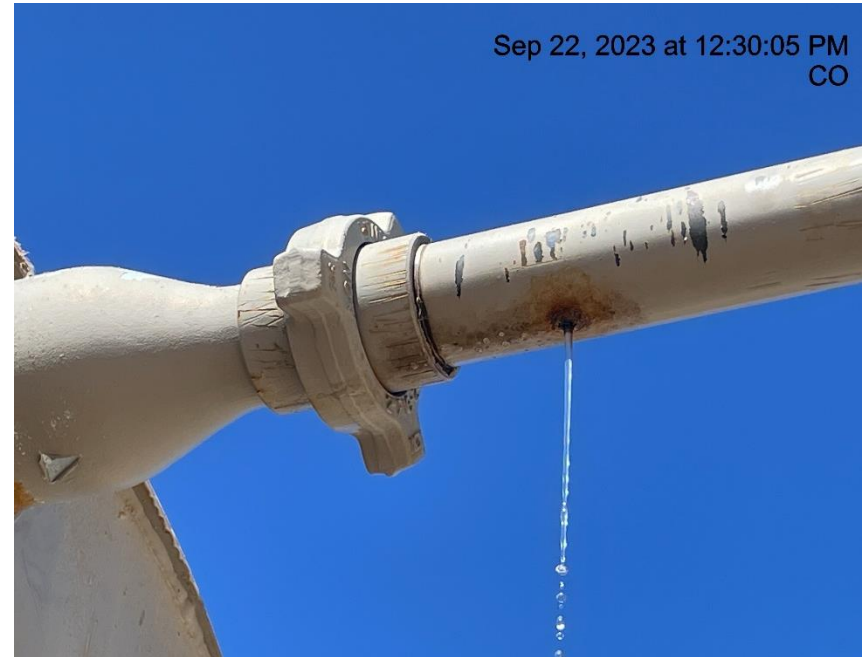
Photo # 494 Hole in production tank flowline & fluid leaking out
