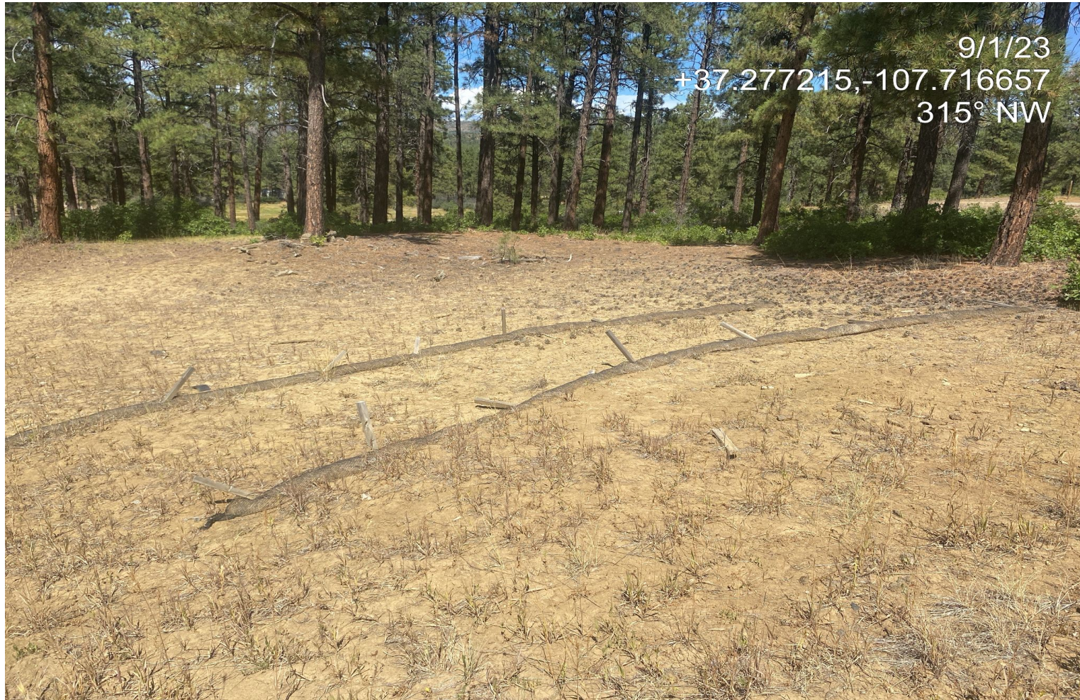
Photo 5. Overview of the northwestern edge of the disturbance. Numerous wooden stakes and wattle BMP's that need to be removed.
