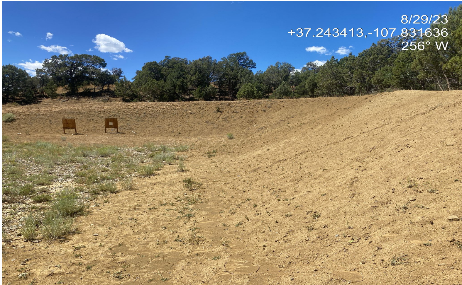
Photo 3. View of cut slope on northern edge of disturbance. Cut slope remains unstabilized with little to no vegetation establishment.
