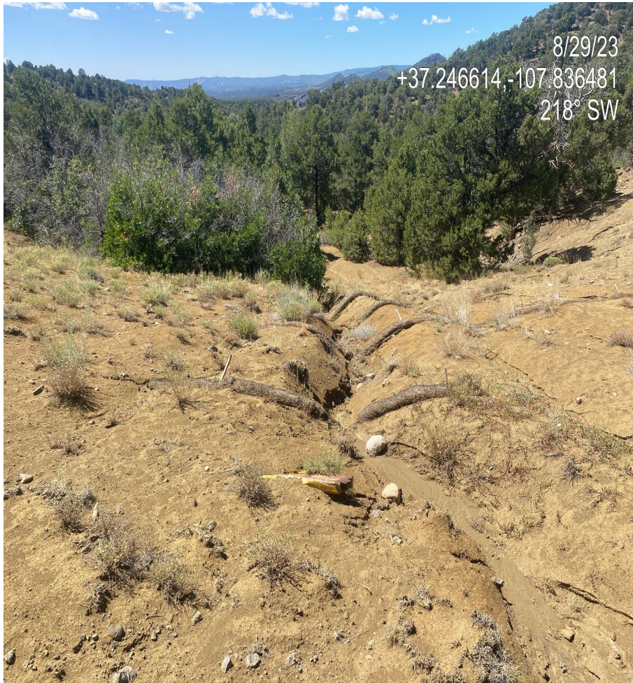
Photo 4. Down and upslope views of erosional channel deepening in southwest corner of disturbance. Currently BMPS are not sufficient for this area.
