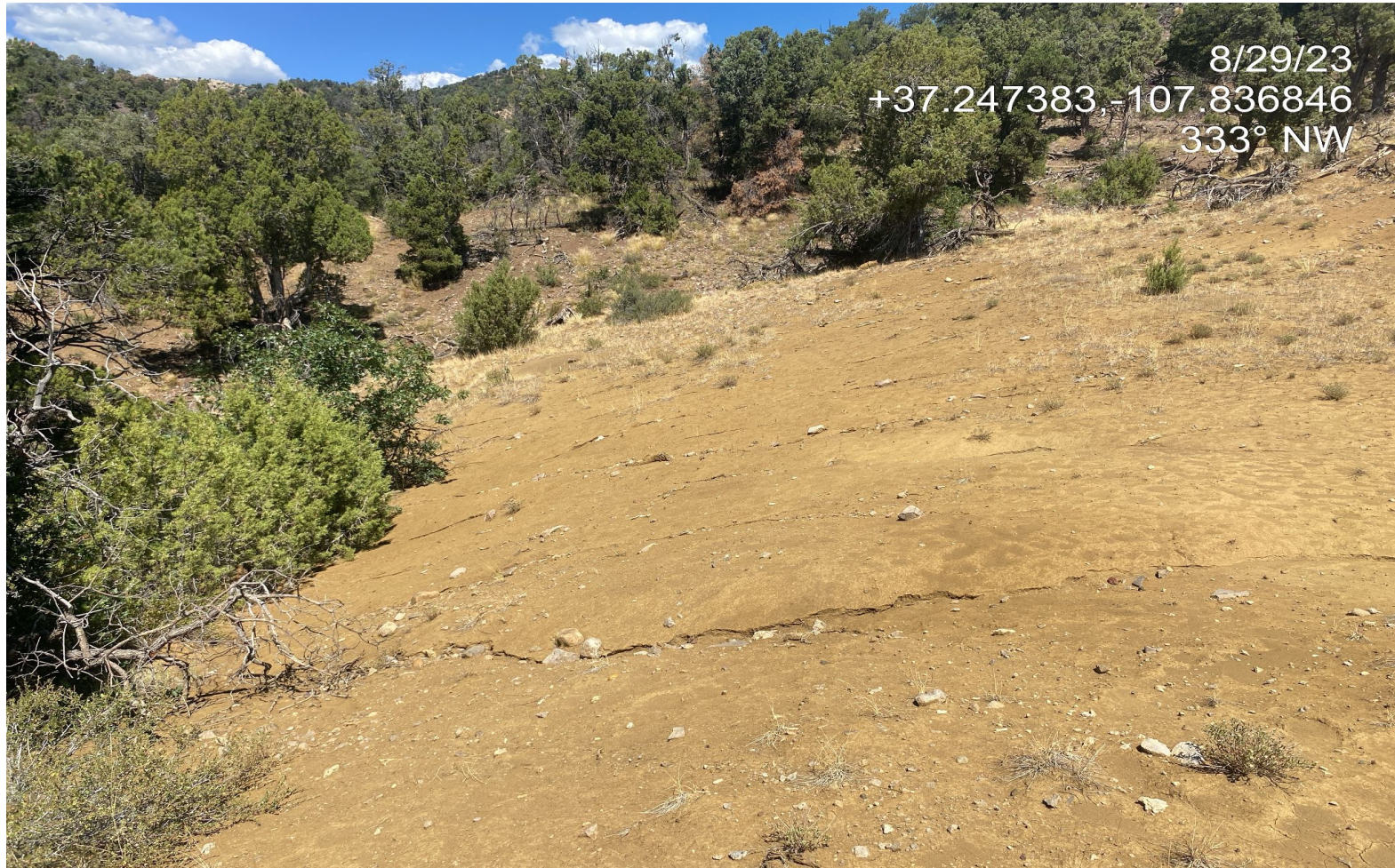
Photo 2. View of the northern project area back slope that has sparse vegetation and rill erosion. Stabilization required in this area.
