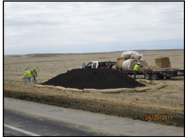
Erosion Logs used for stockpile management practices
