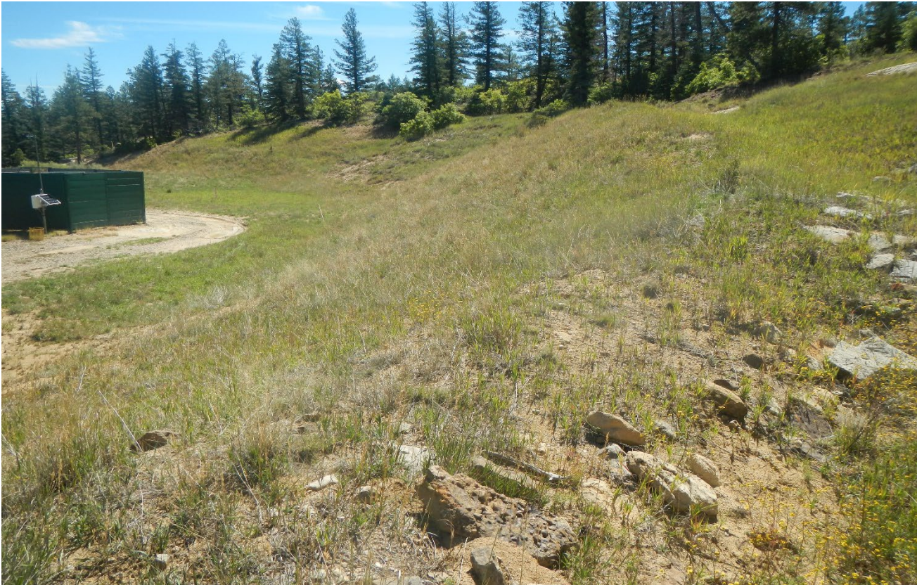
Photo 2. Facing east toward the cut slope which is stabilized with vegetation.
