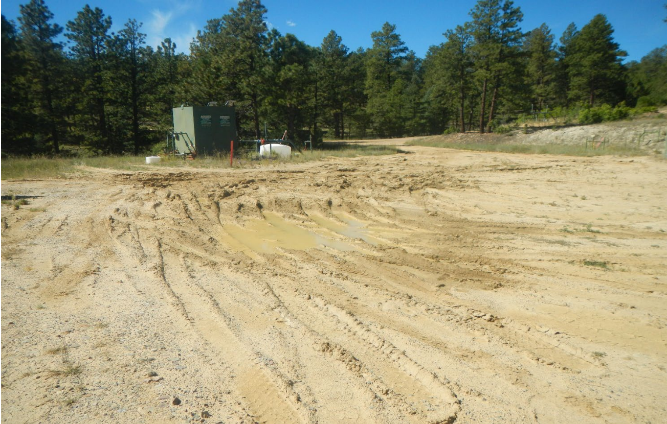
Photo 3. There is vehicle rutting at the location which is not stabilized.
