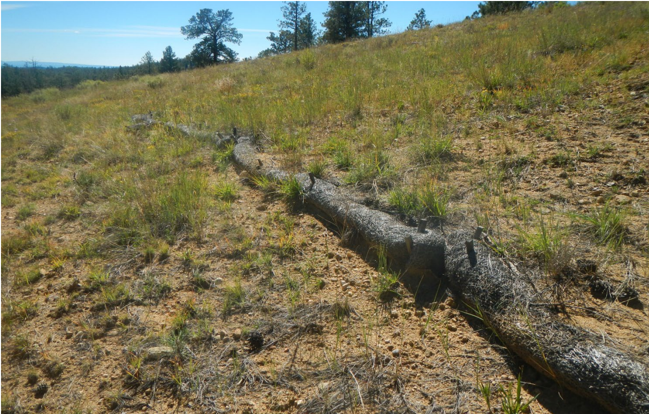
Photo 6. The stormwater wattles will need to be removed prior to final inspection.
