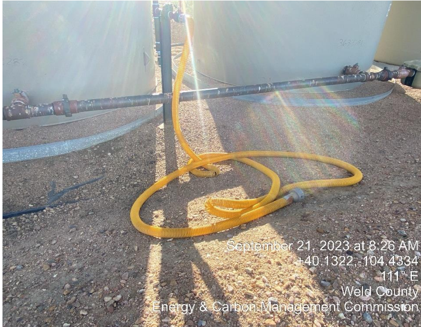
Weathered/ Ripped Vapor Line hose
