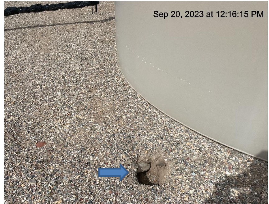
Photo # 26 Hole in base of secondary containment
