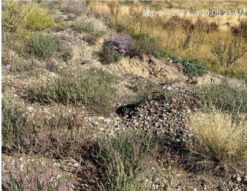
Berm erosion remains unchanged from May 2023 inspection
