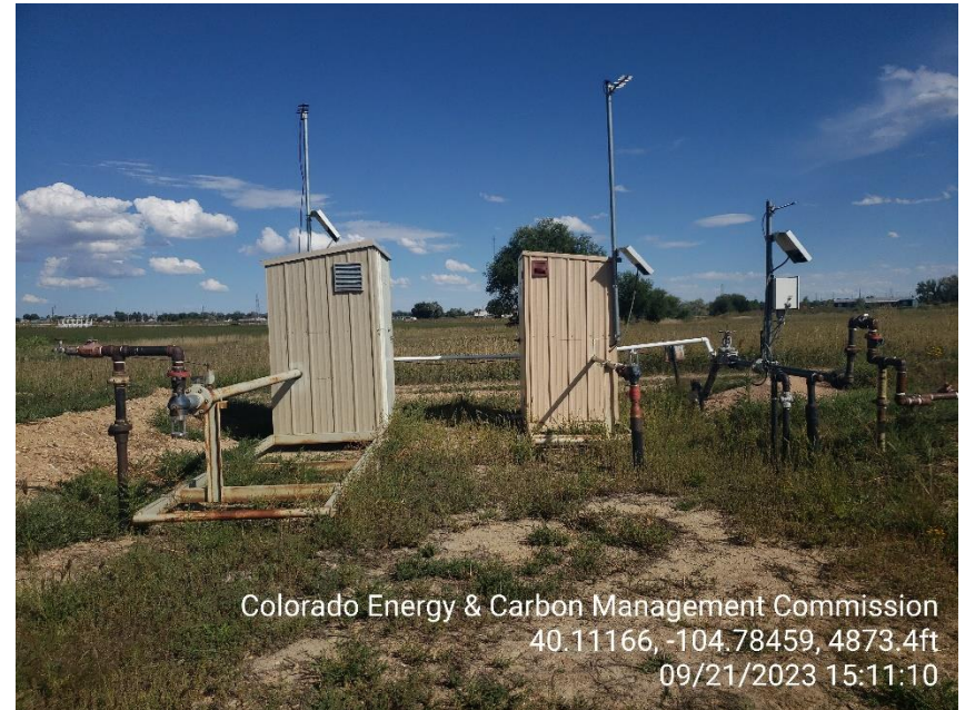
Photo 8 Gas Meter Run.
