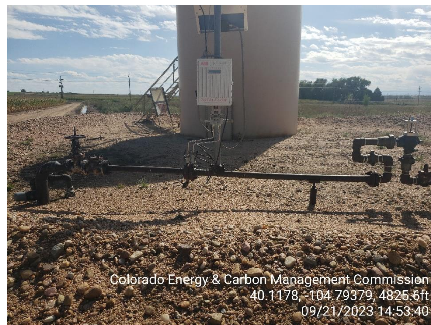
Photo 4 Gas Meter Run.
