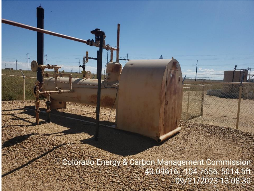
Photo 7 Horizontal Heated Separator.
