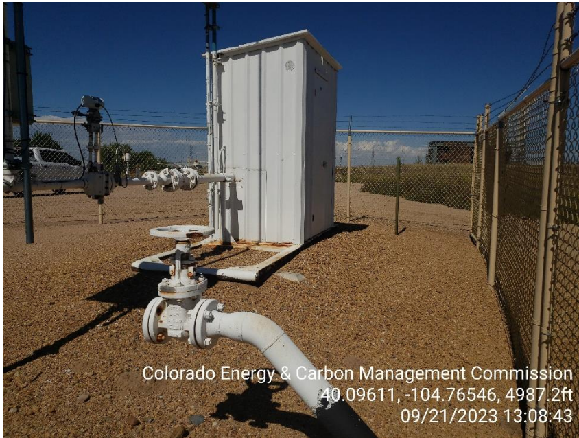
Photo 3 Gas Meter Run.
