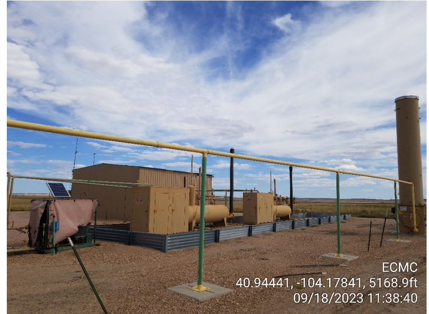
Photo 4 – Separators, VRU and ECD
