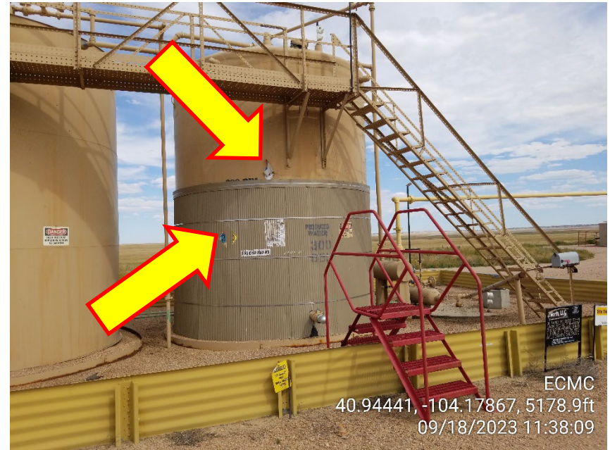
Photo 2 – NFPA Label faded no longer visible
