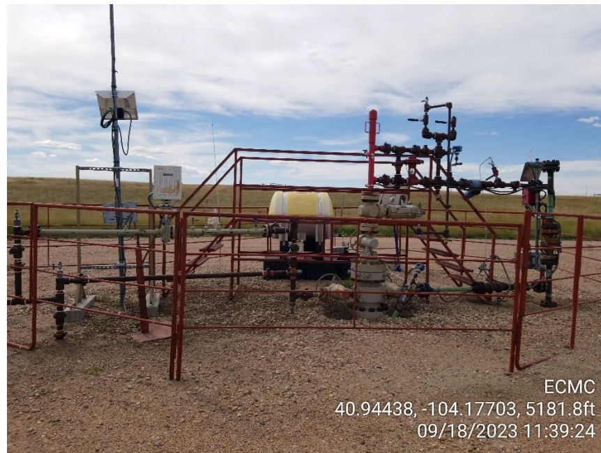
Photo 6 – Wellhead – Chemical Tank missing label
