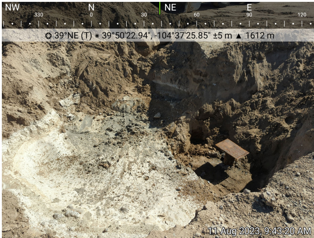
Photo 1: DIA #35-11 P&A wellhead excavation, 8/11/2023.
