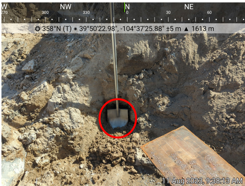
Photo 2: SS01 collected from P&A wellhead excavation, 8/11/2023.
