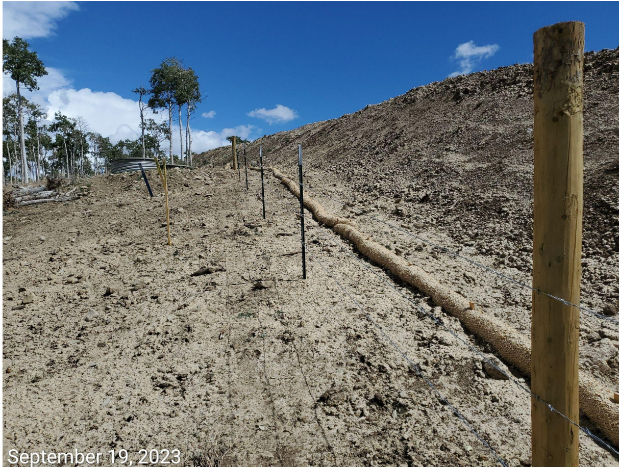
Photo 7: Photo taken from the northern perimeter of the Location's disturbance area. Photo shows Operator has implemented an erosion log to minimize off-site sediment transport in conjunction with hydromulch.
