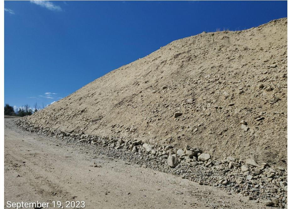
**Photo 1:** Photos taken from the tow of the fill slopes on the northeast and east end of the Location. Photo shows Operator has implemented hydromulch on the slopes. Control measure appeared to be in proper functioning condition at time of inspection.
