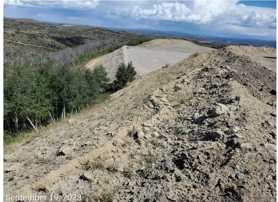
**Photo 3:** Photo left taken from the interim areas on the southwest end of the Location. Operator appears to have conducted additional reclamation work in conjunction with a hydromulch application. Photo right also shows erosion logs have been maintained.
