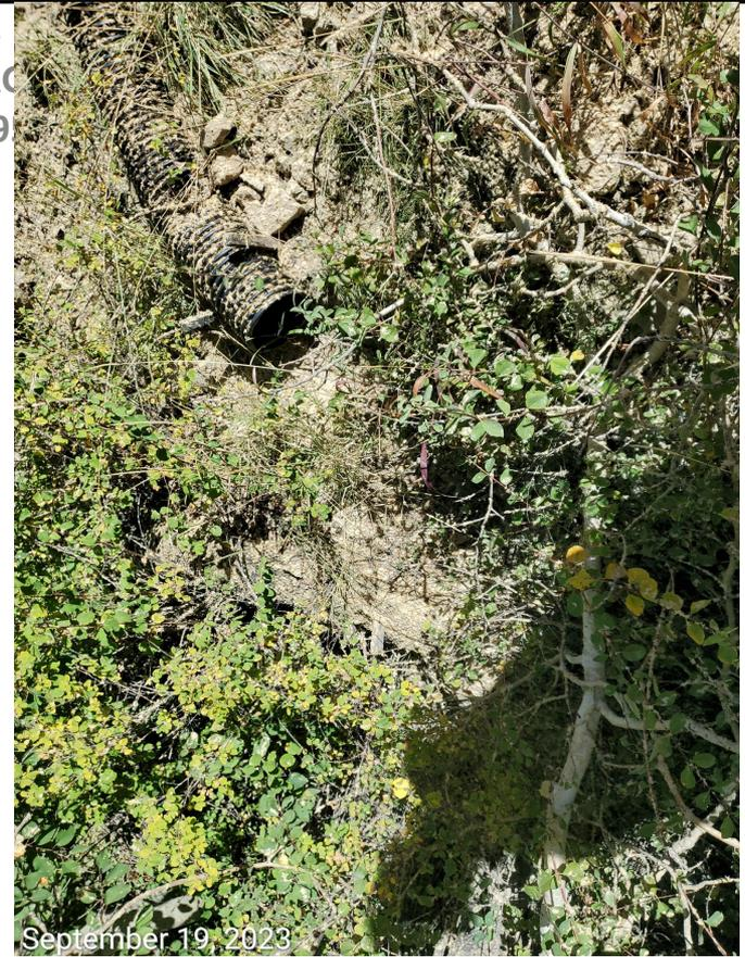
**Photo 4:** Photo left shows the outlet from the working pad surface has been maintained and sediment removed. Photo right shows the slope drain outlet lacks a properly engineered and armored outlet, resulting in off-site degradation.
