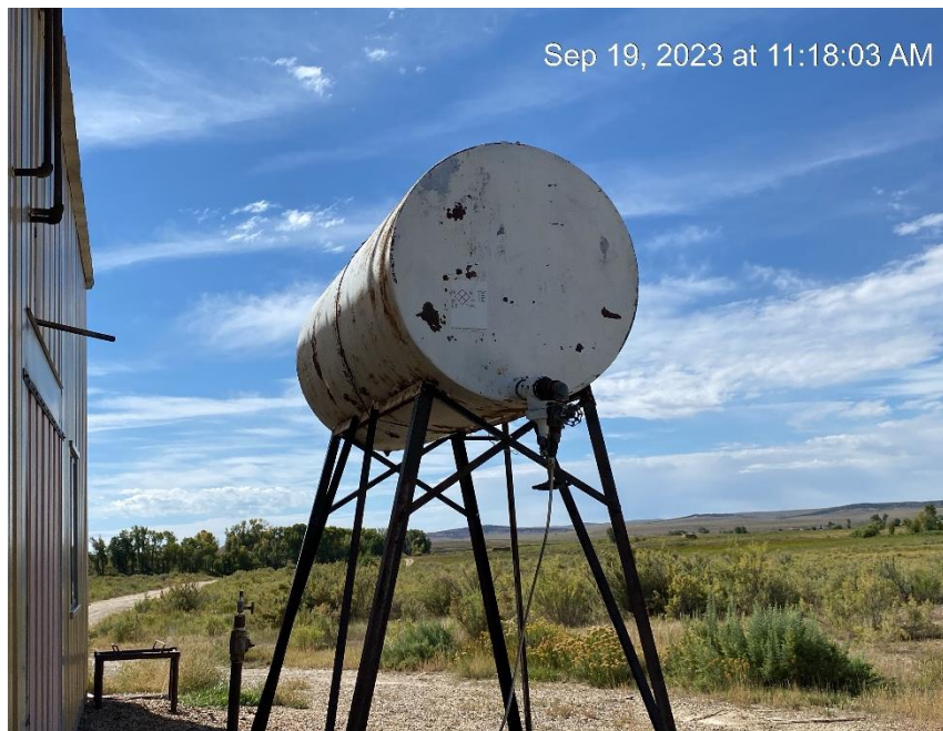
Unlabeled tank, no containment
