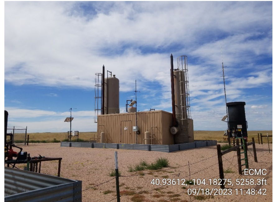
Photo 4 – Heater Treaters and ECD
