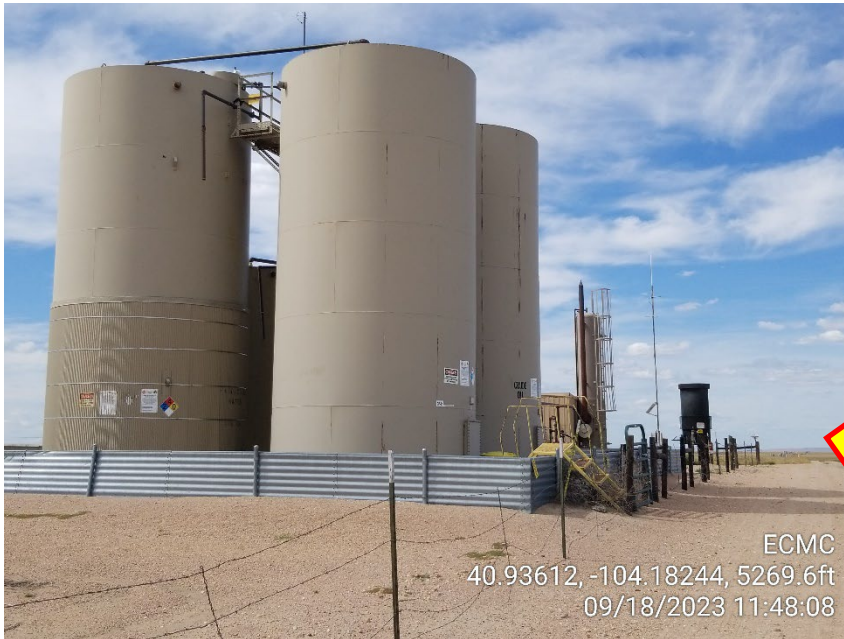
Photo 1 – Tank Battery
