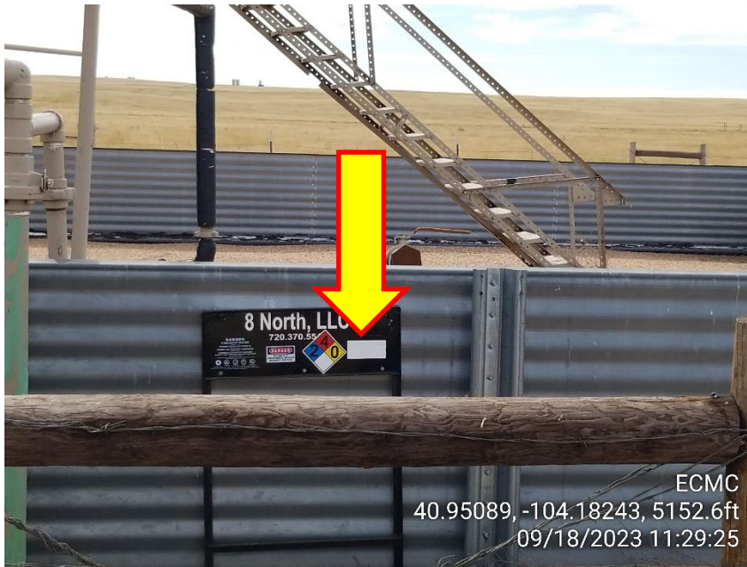
Photo 3 – Missing Capacity Label
