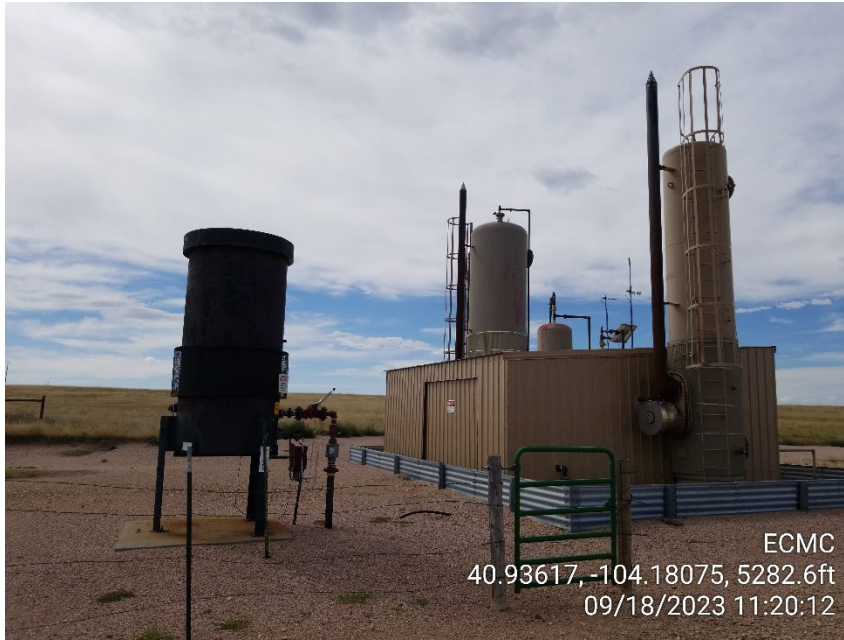
Photo 1 – ECD and Heater Treaters
