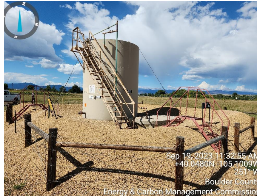
Photo 4 tank battery
