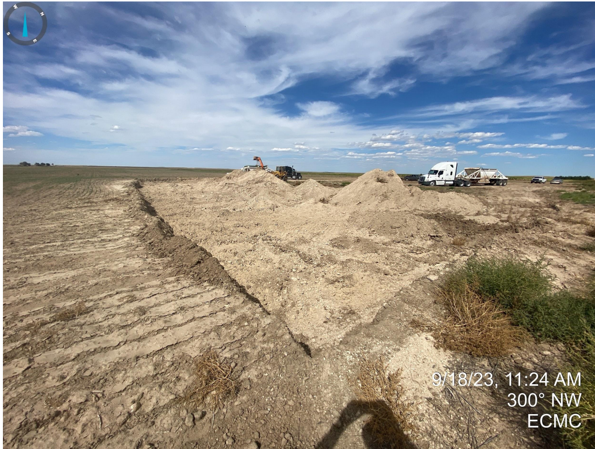
Photo 2. Taken from the southeast corner of the former pit. Photo illustrates excavation operations of E&P waste occurring over the former pit. Onsite Operator representative informed Staff that the waste was being sent to Washington County Landfill for disposal.
