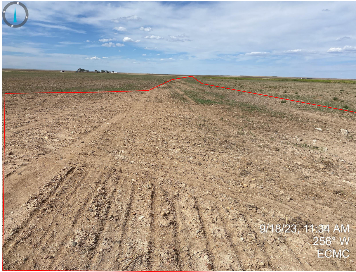
Photo 6. Taken north of the former production areas. Photo illustrates that road base/gravel remains throughout the northern portion of the production areas and along the former access road to the wellhead. Final reclamation activities are required.
