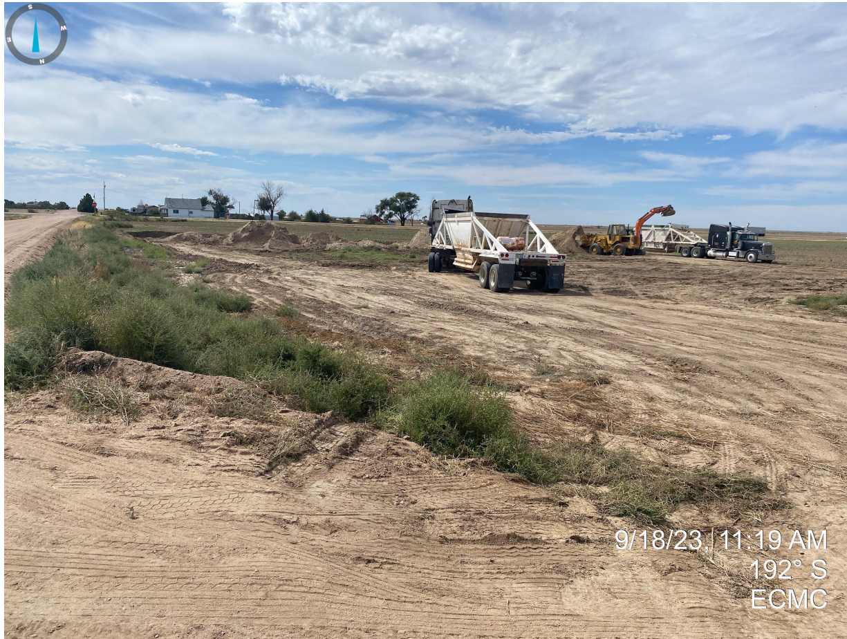
Photo 1. Taken at the location's entrance. Photo illustrates excavation operations (digging and hauling) of the former pit area.
