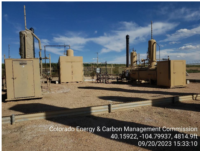
Photo 3 Horizontal Heated Separators & Vertical Separators.
