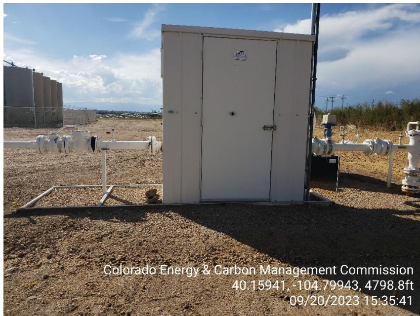
Photo 5 Gas Meter Run.
