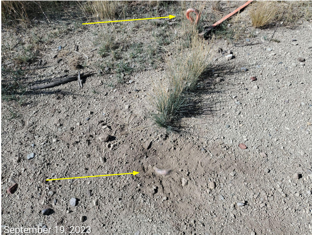
Photo 7: Photo shows two unmarked anchors on the southern working pad surface.
