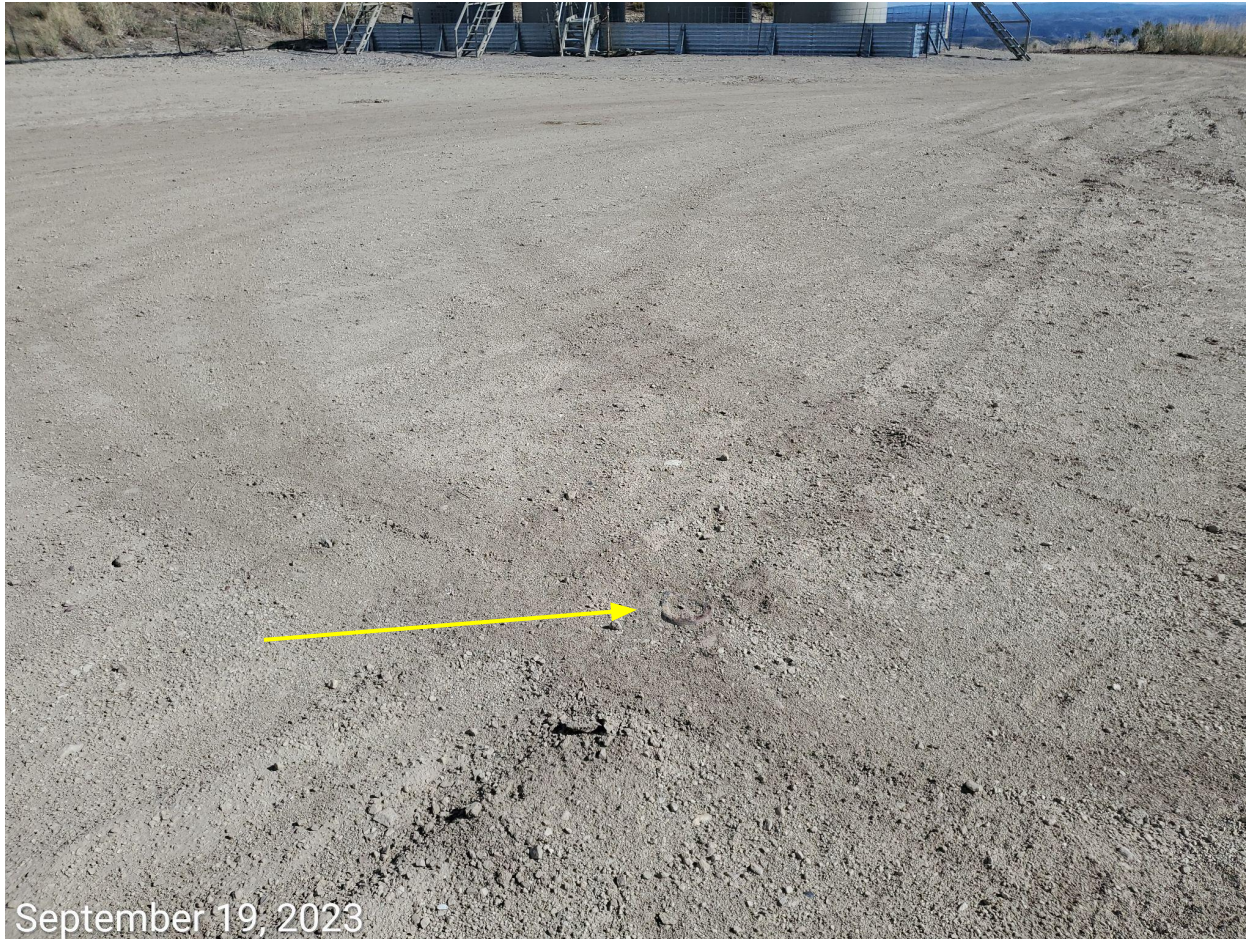
Photo 9: Photo shows unmarked anchor on the eastern working pad surface.
