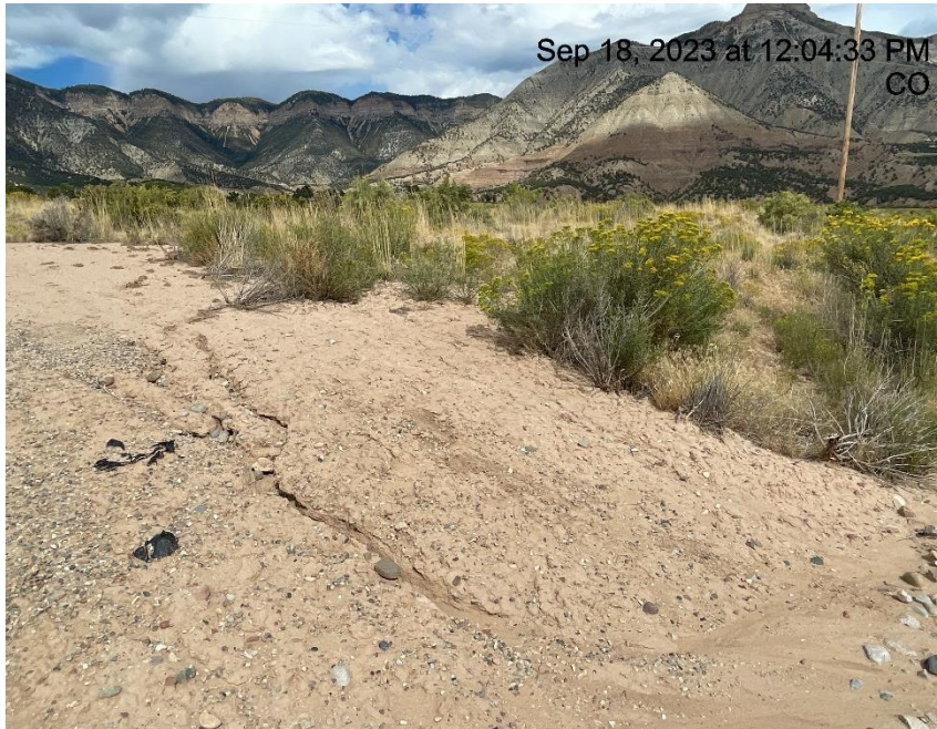
Photo # 9733 Erosion & transport of sediment off location/insufficient BMP's
