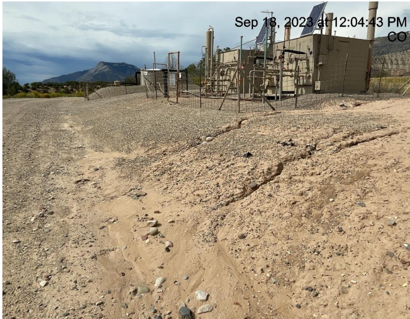
Photo # 9735 Erosion & transport of sediment off location/insufficient BMP's
