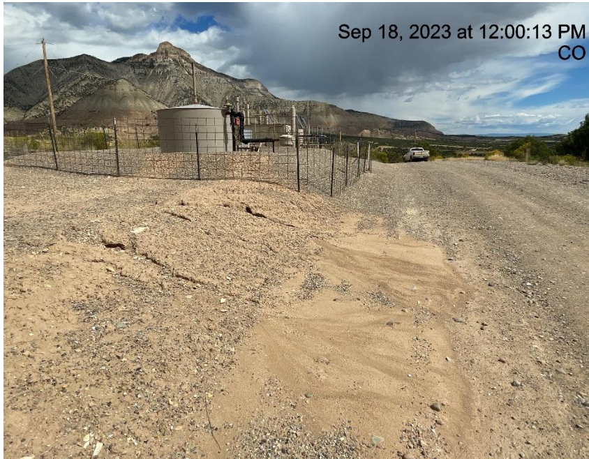
Photo # 9709 Erosion & transport of sediment off location/insufficient BMP's
