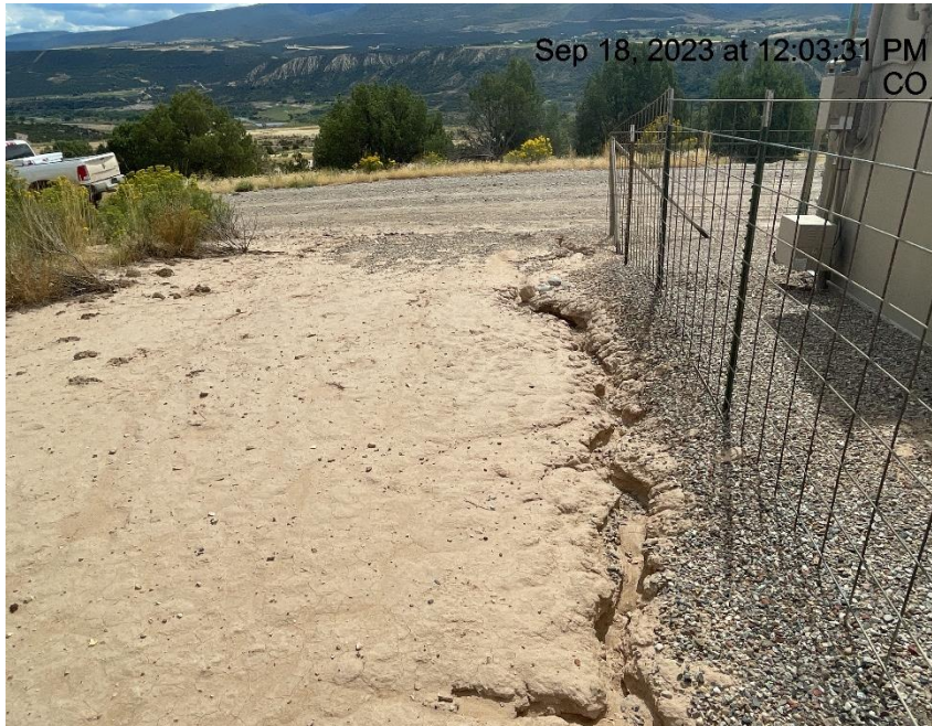
Photo # 9724 Erosion & transport of sediment off location/insufficient BMP's
