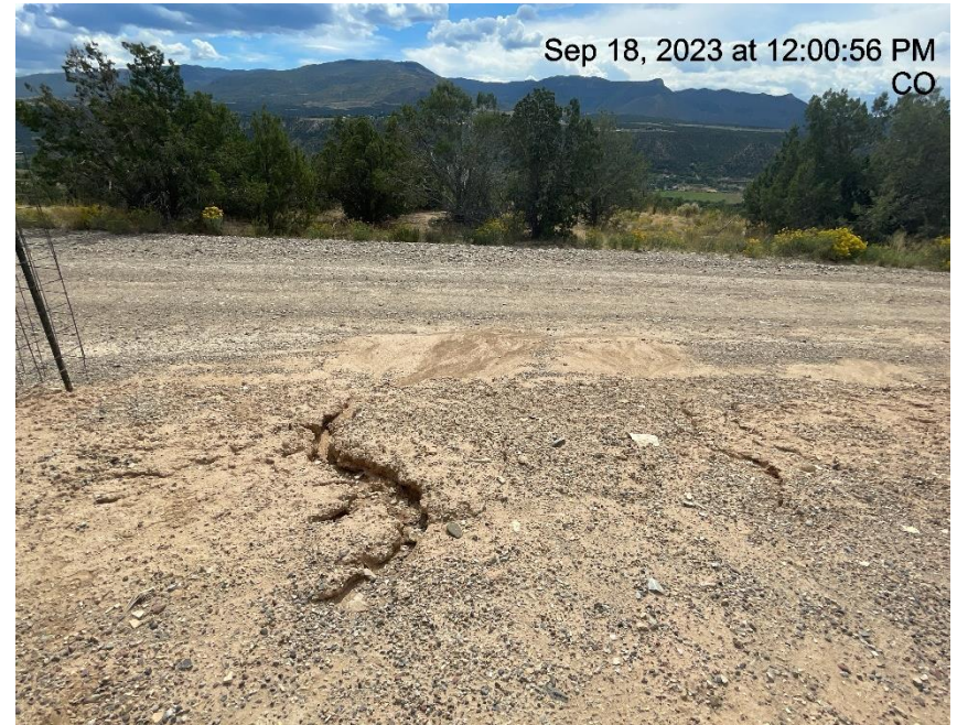
Photo # 9716 Erosion & transport of sediment off location/insufficient BMP's
