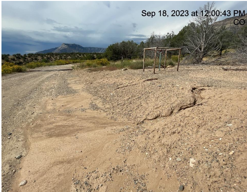
Photo # 9715 Erosion & transport of sediment off location/insufficient BMP's
