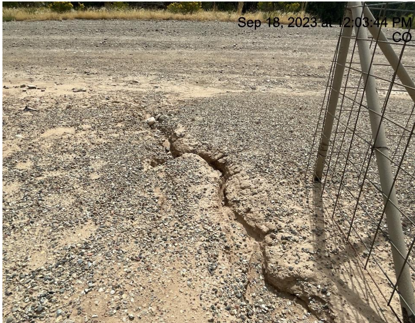
Photo # 9726 Erosion & transport of sediment off location/insufficient BMP's
