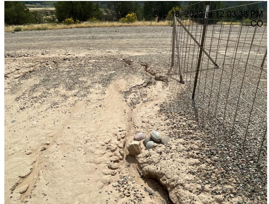
Photo # 9725 Erosion & transport of sediment off location/insufficient BMP's
