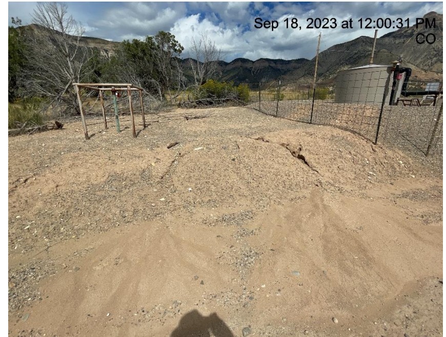
Photo # 9712 Erosion & transport of sediment off location/insufficient BMP's
