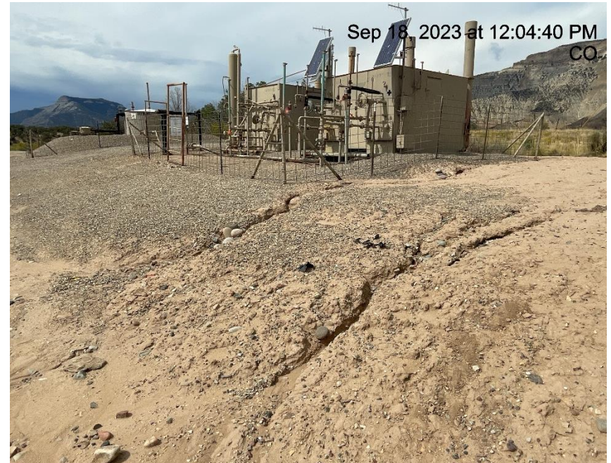
Photo # 9734 Erosion & transport of sediment off location/insufficient BMP's
