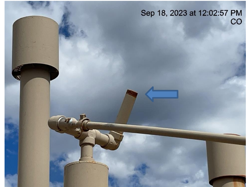
Photo # 9721 Open ended pipe/wildlife hazard
