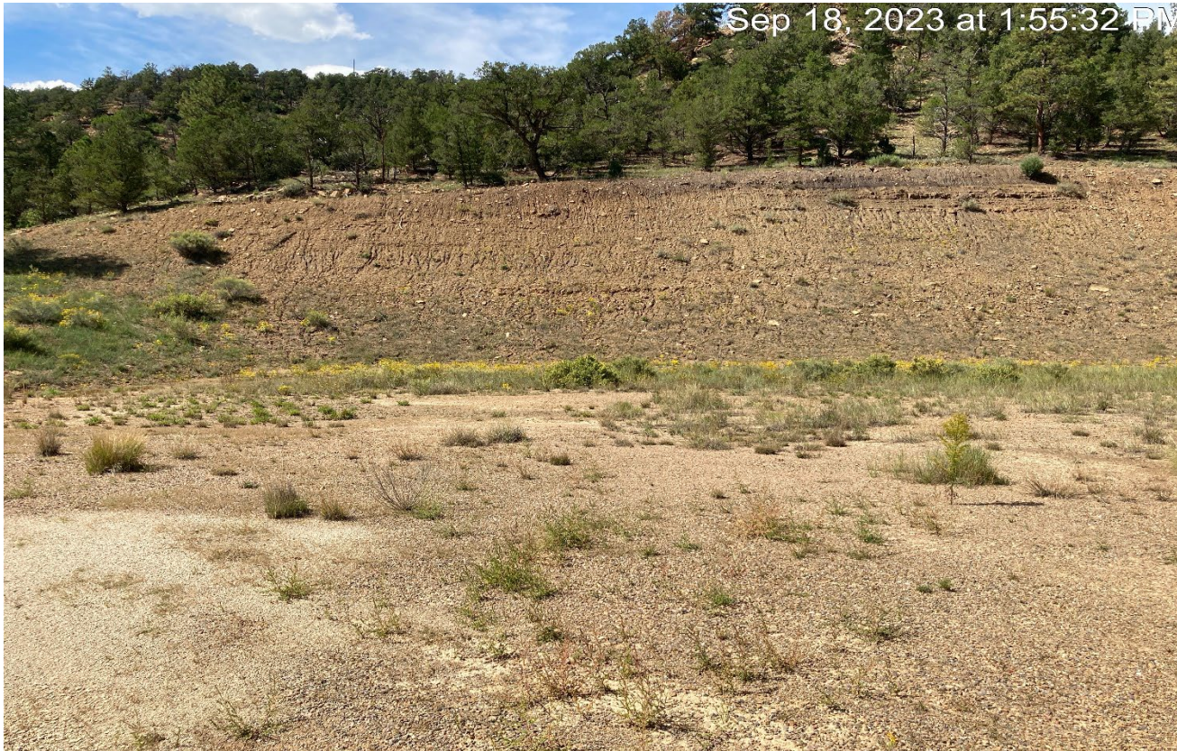
Photo 6. Center of the location facing west toward the cut slope. There are signs of erosion along the cut slope which is not stabilized.
