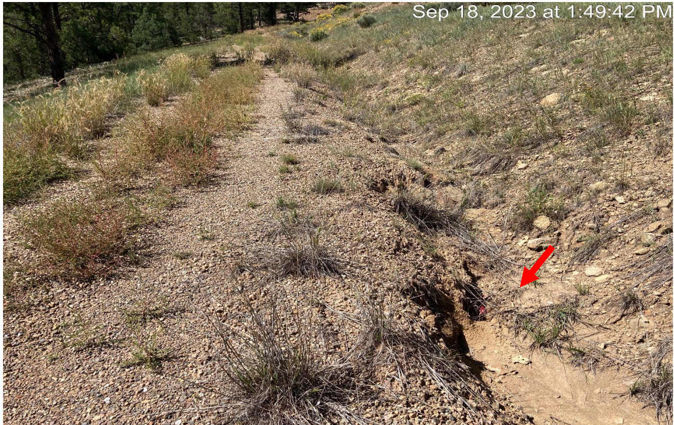
Photo 2. Facing northwest along the access road. There is erosion at the red arrow that will require BMP's for stabilization..
