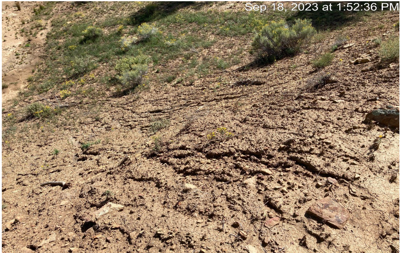
Photo 10. View of erosion occurring along the cut slope..
