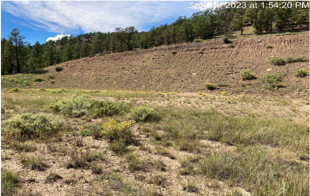
Photo 8. Facing southwest toward the cut slope. There are signs of erosion along the cut slope which is not stabilized.
