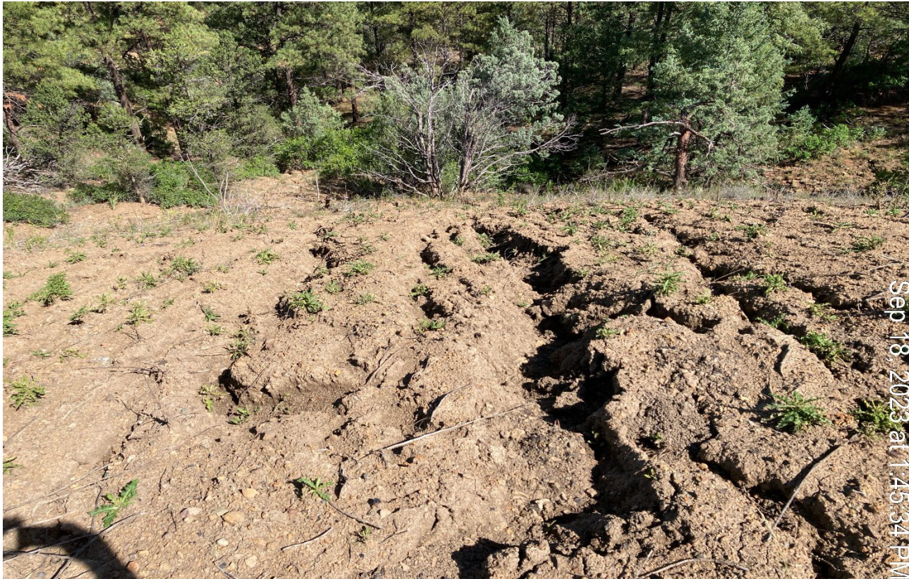
Photo 4. There is erosion along the fill slope that needs to be repaired and stabilized.
