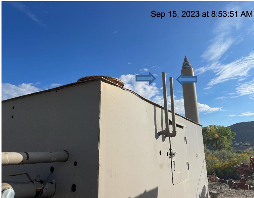
Photo # 9441 PRV vent & rupture disc vent lack caps
